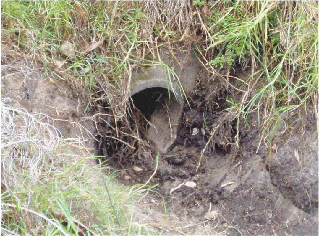
Figure 2.5 Outfall 5 directly discharging into Lake Joondalup via a channel (Photo source: author).
