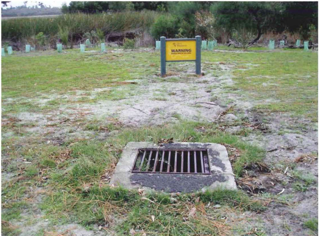
Figure 2.6 Bubble up grate 2 showing indirect inputs to Lake Joondalup (Photo source: author).
