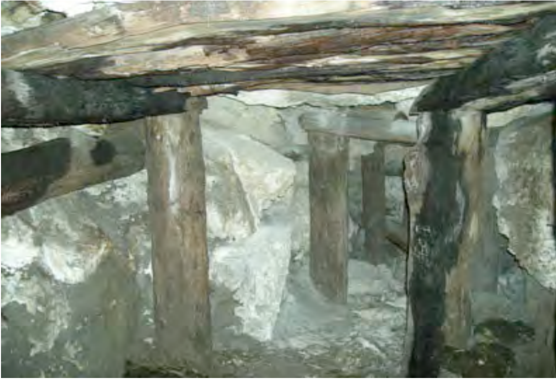
Figure 31: Caves on the northwest shores of Lake Joondalup excavated by early settlers to drain water from Lake Joondalup through a labyrinth of caves to the sea.
