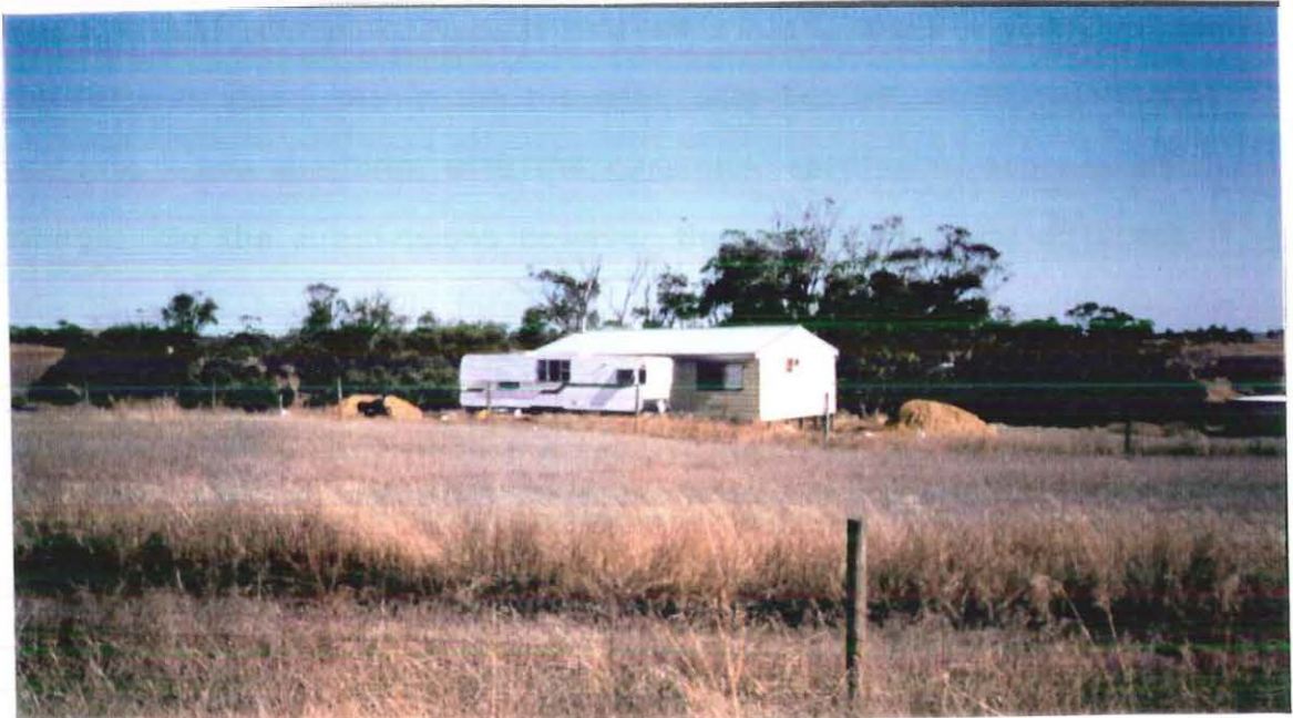
Plate 5:2 This unfinished dwelling is typical of many found on the inland subdivisions. In contrast with the Rolling Green estate, these houses are often smaller and built to a much lower cost. The caravan in the Plate was being used as temporary accommodation while the dwelling was under construction.
