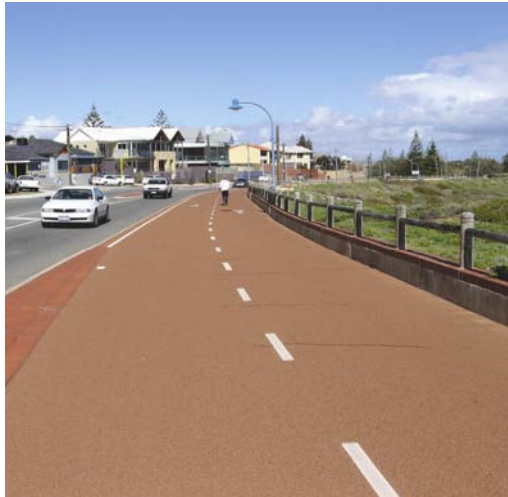
Figure 4.2: Initial portion of Route 1
