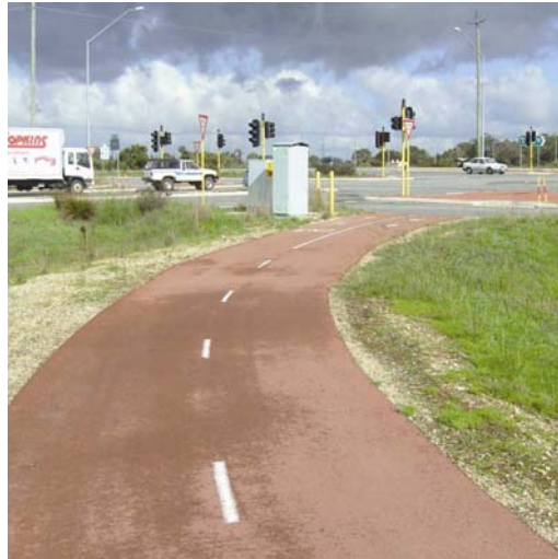
Figure 4.18: Road crossing on Route 3
