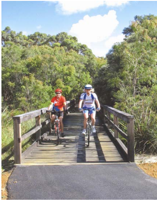
Figure 2.34: Cycling bridge on a paved route (Courtesy of Tourism WA)
