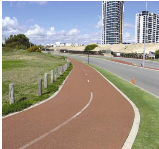
Figure 4.23: Initial portion of Route 4
