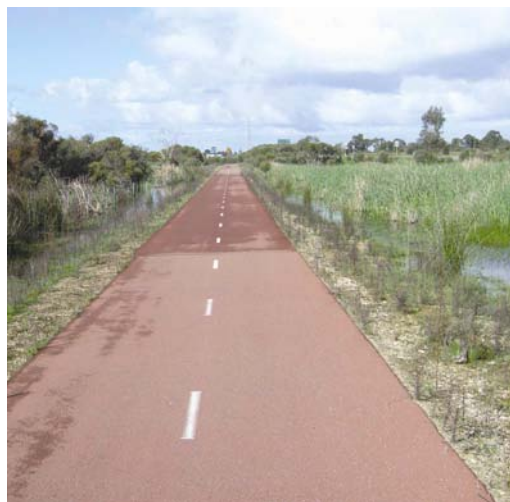
Figure 4.20: Path crosses swamp land near the end of Route 3
