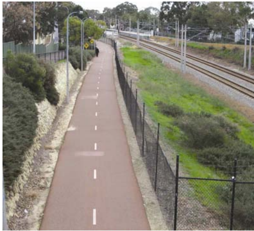
Figure 4.9: Initial portion of Route 2
