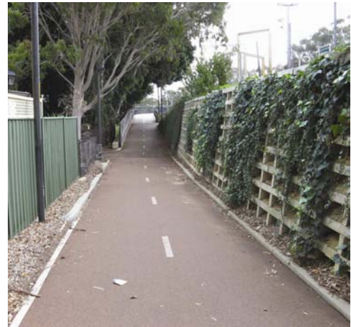
Figure 4.10: Initial portion of Route 2
