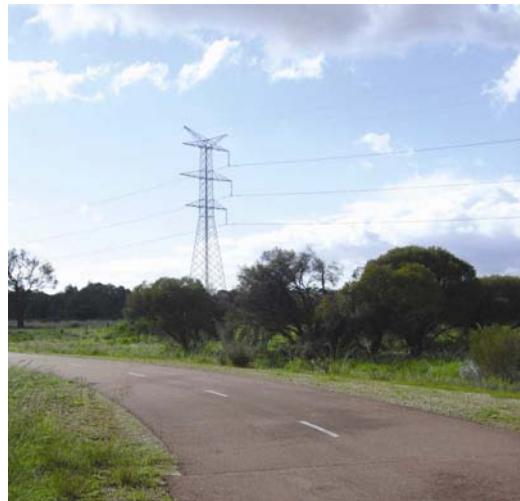
Figure 4.17: Electrical pylons in the vicinity of Route 3
