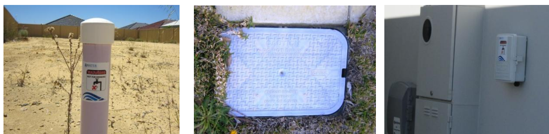
Figure 12: The labels of NDG system at the connection point, filter box, and controller
