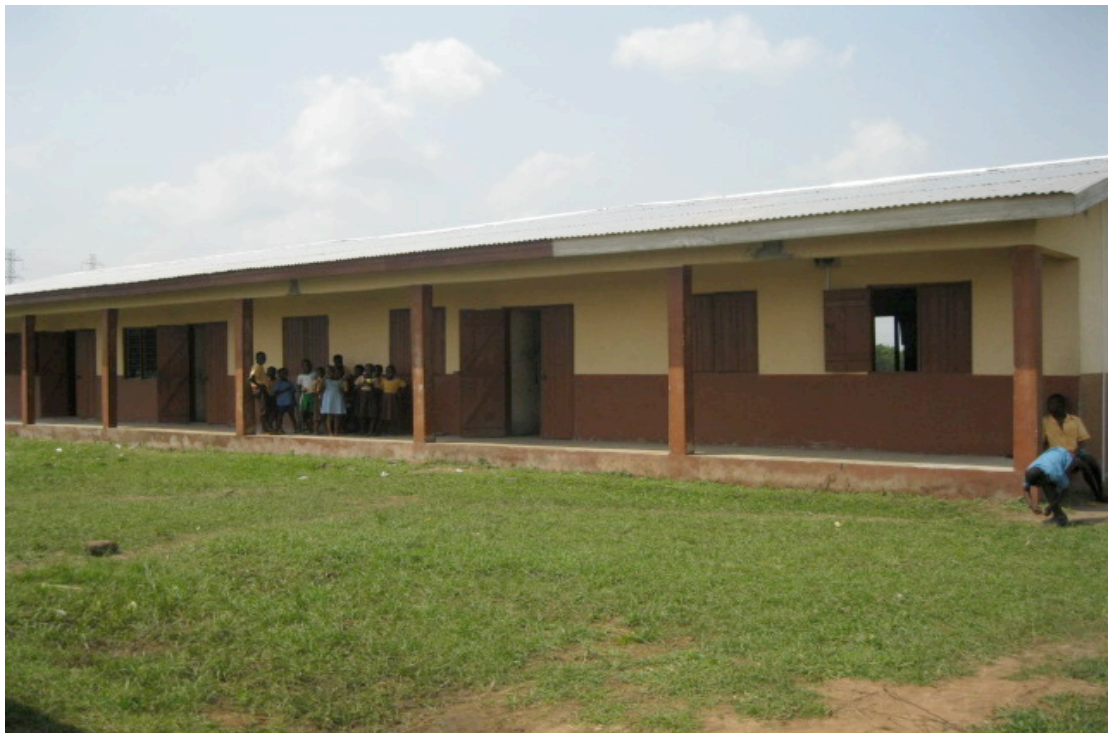
Photo 6.6: The Agbetor CBRDP Three-Unit Classroom Block.
