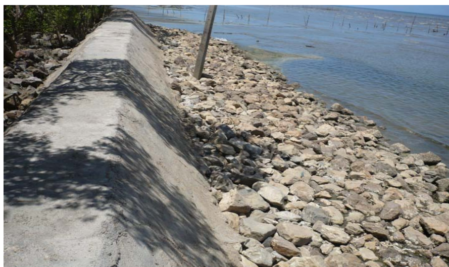
Figure 4-4. A seawall in the low erosion area
