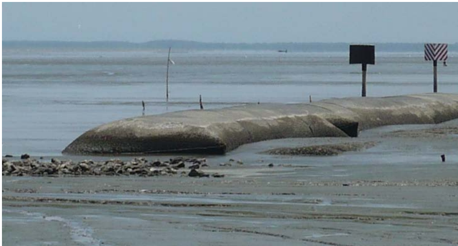
Figure 4-2. Sand tubes were installed in a low erosion village.
