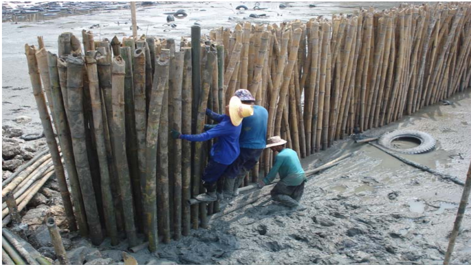
Figure 4-8. Bamboo stems were embedded in the sea floor to protect coastal areas Source: The Coastal Conservation Networks in the upper Gulf of Thailand, 2010
