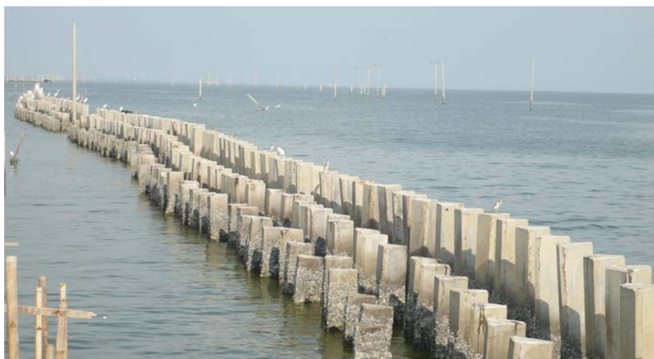
Figure 4-5. Embedded triangular poles in the sea bed offshore to protect coastal area
