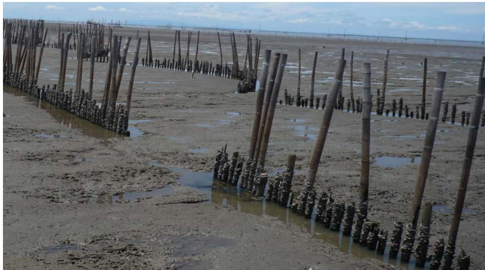
Figure 4-6. Bamboo stems were decayed and broken.
