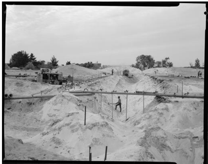
Figure 45. Millars Dewatering system at an excavation, 1965.
