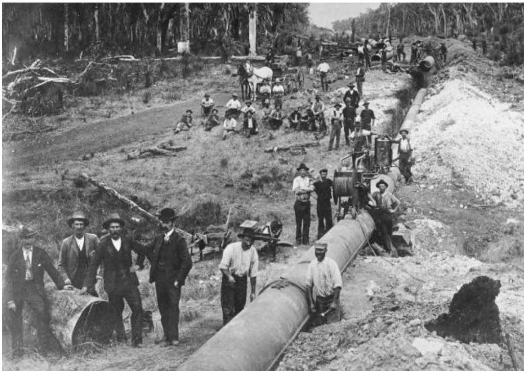
Figure 47. Laying the Golden Pipeline from Perth to Kalgoorlie.
