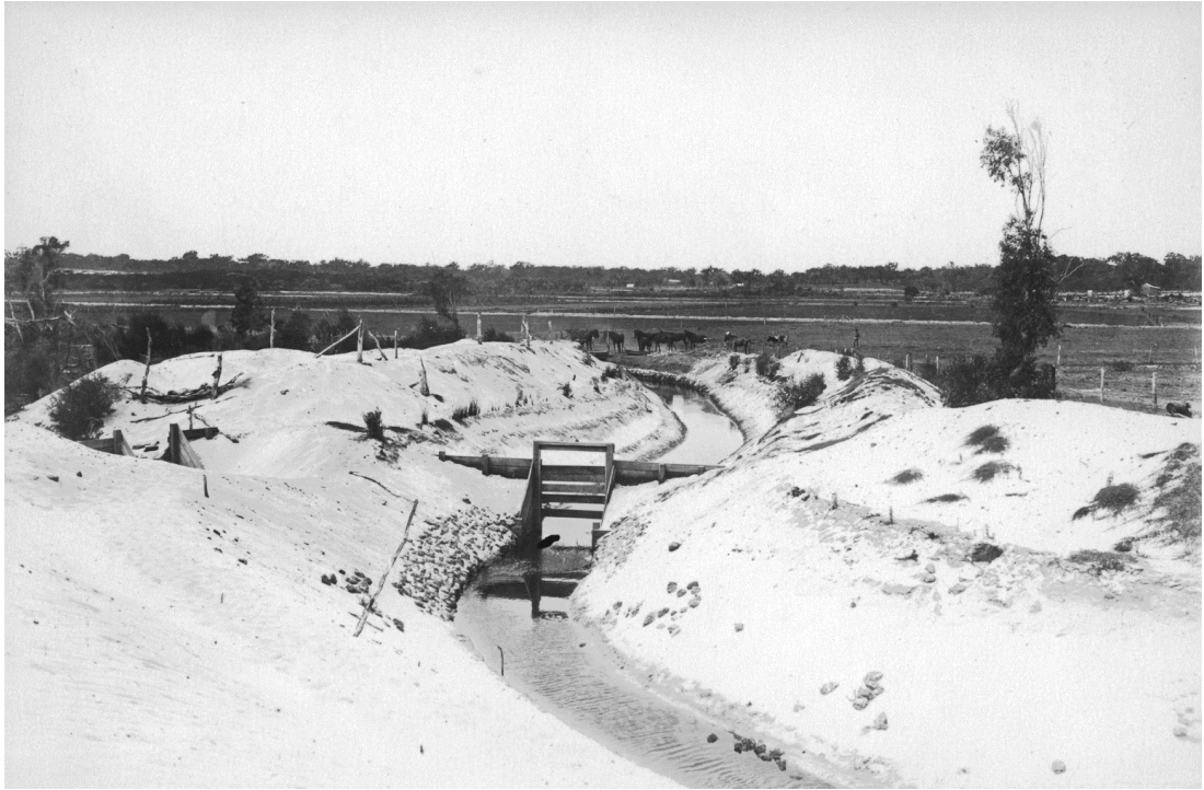
Figure 42. Drain and general view of reclaimed swamp 1920s. Image courtesy of the State Library of Western Australia, 006733d. (Exception to copyright ss40, 103C; research or study).
