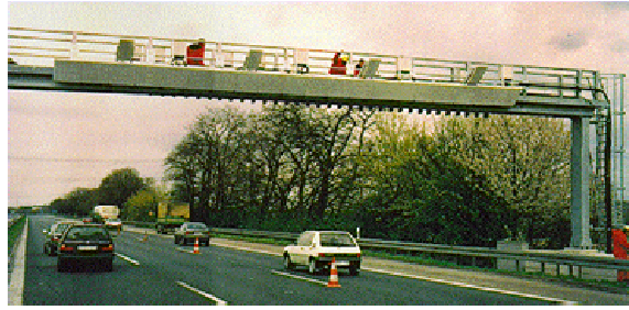
Figure 2.5: DSRC used for toll collection
