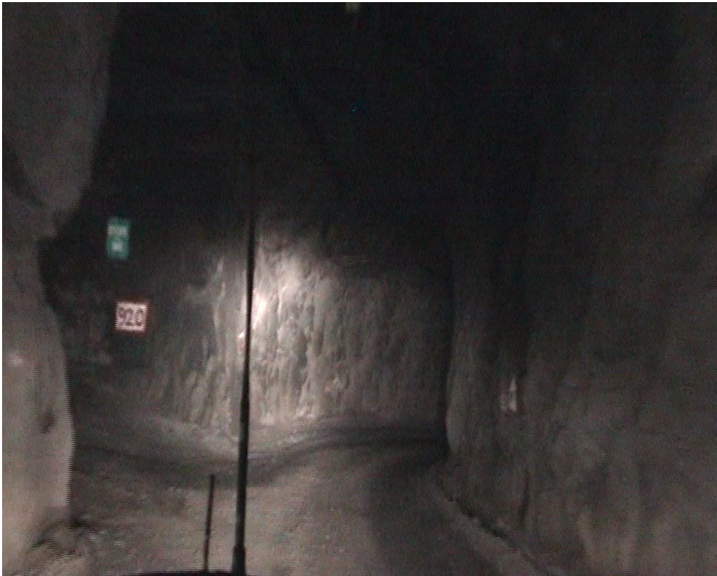
Figure 4.5. Examples of depth level and reflective green escape rise signs within the Challenger mine
