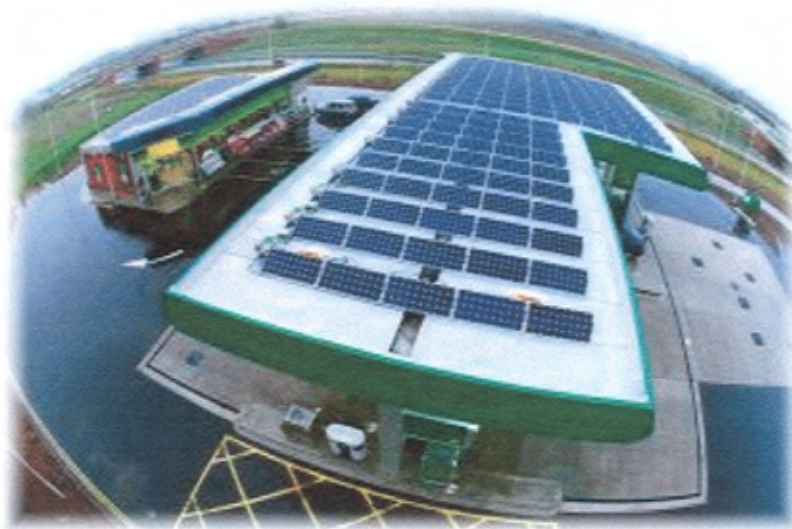
Figure 4-9 Example of non-domestic roof PV system (Source www.pv-uk.org.uk )
