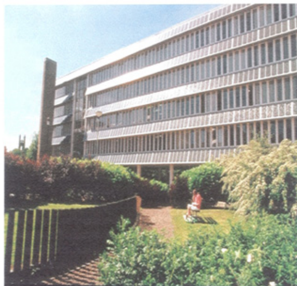
Figure 4-12 Northumberland Building PV façade system at Northumbria University, Newcastle upon Tyne
