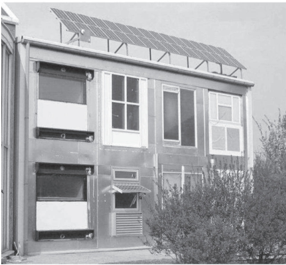
Figure 4: Fraunhofer ISE façade testing facility. The test offices are the two rooms at the left hand end of the building (Schossig et al, 2005).
