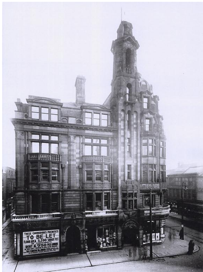
Figure 19 Pearl Assurance building, Northumberland Street c.1930, designed by William Hope, 1904. (Newcastle City Library).
