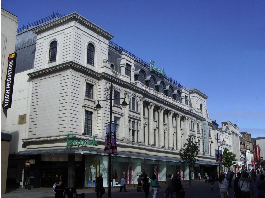
Figure 12 Fenwick's, Northumberland Street. (Author's photograph).
