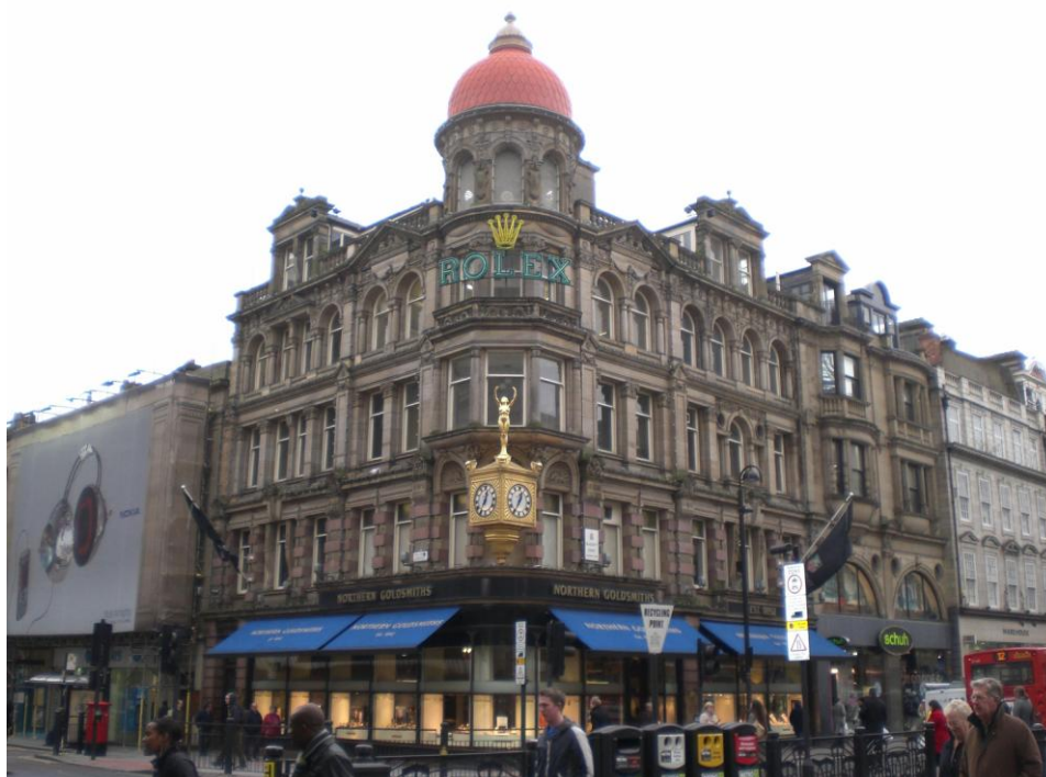
Figure 125 Northern Goldsmiths' Building, Nos. 1-7 Blackett Street, designed by James T. Cackett, c.1890-2. (Author's photograph).
