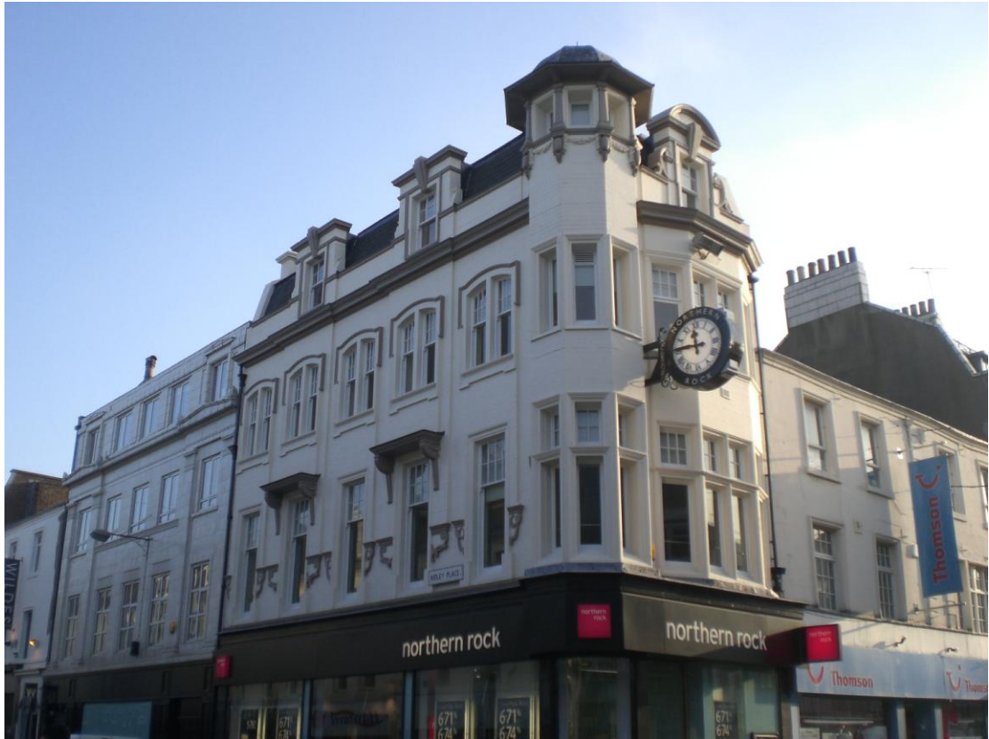
Figure 25 No. 132-134 Northumberland Street. (Author's photograph).
