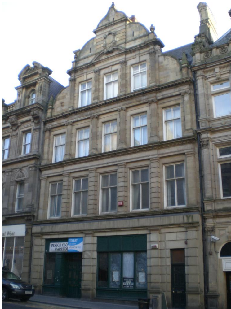
Figure 121 Oxford House, Nos. 34-40 Grainger Street West, designed 1874. (Author's photograph).
