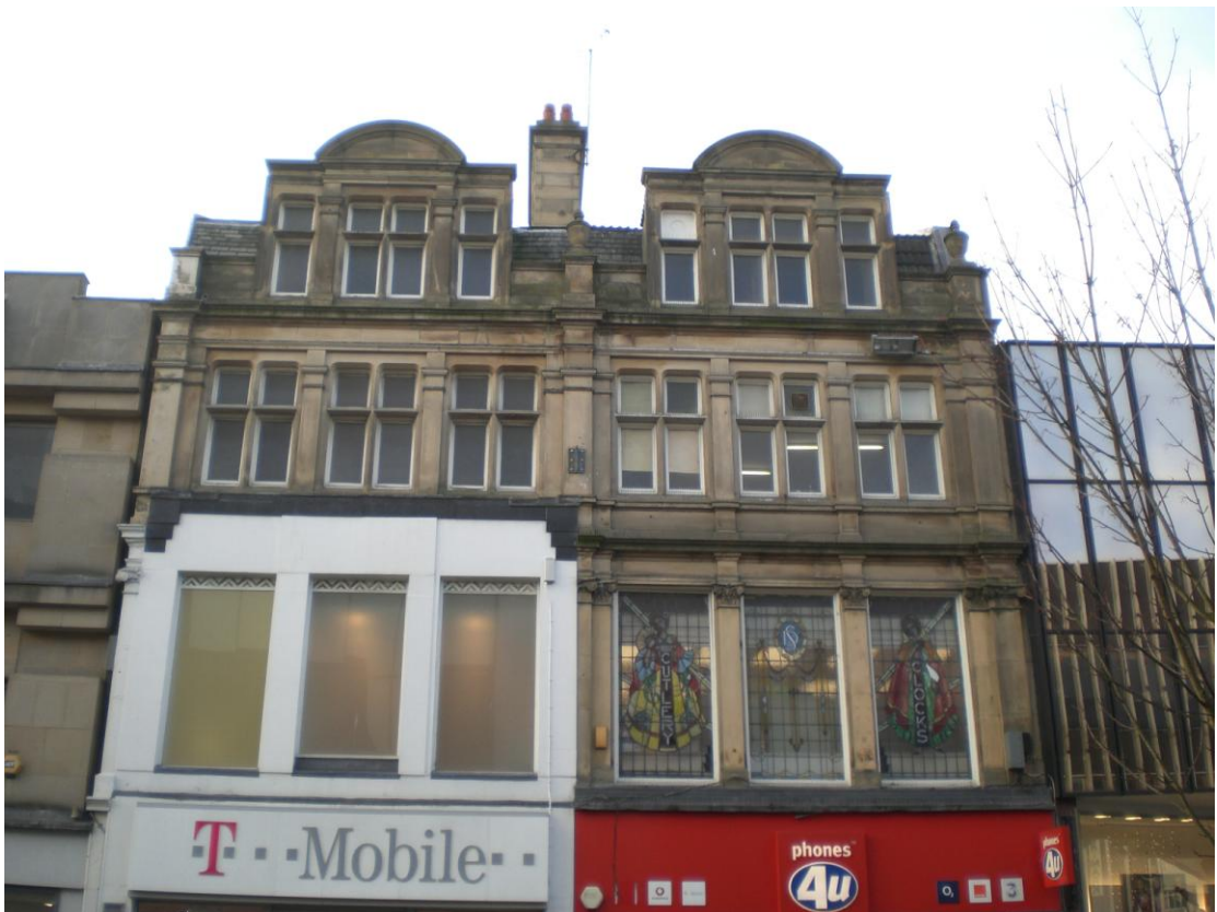
Figure 22 Nos. 61-63 Northumberland Street. (Author's photograph).
