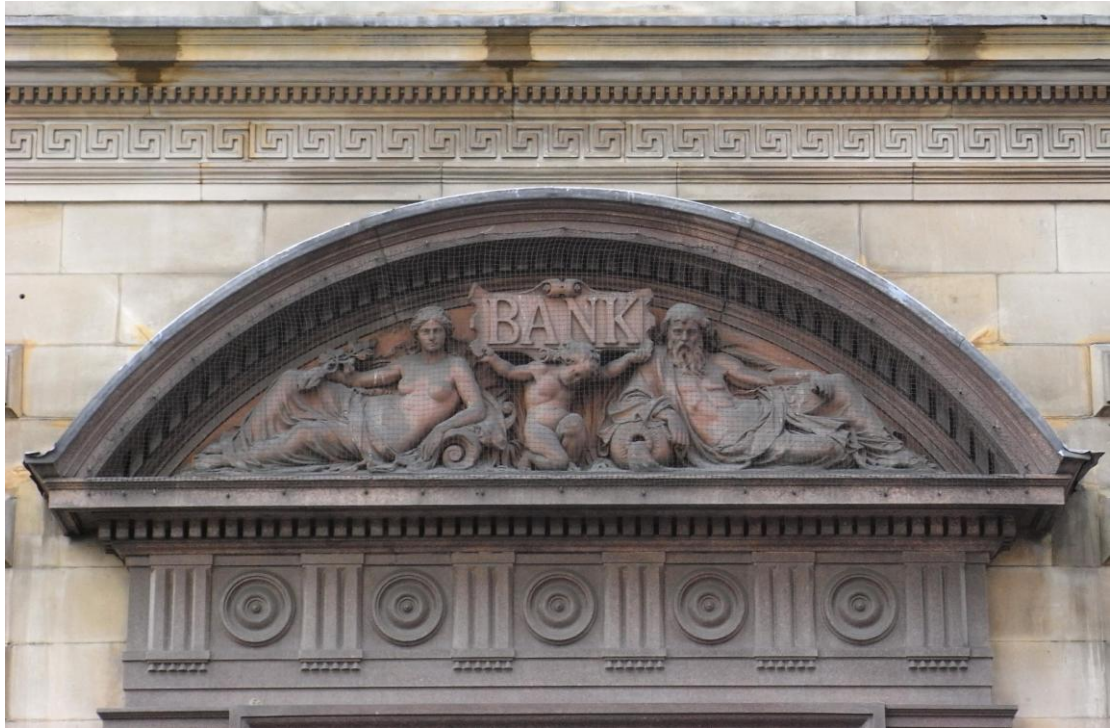
Figure 89 Detail of Hodgkin, Barnett, Spence, Pease and Co. Bank, Collingwood Street, designed by R.J. Johnson, 1888-92. (Author's photograph).
