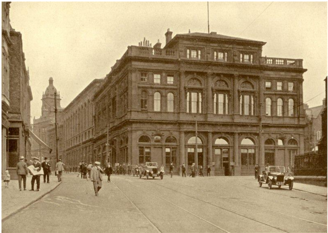
Figure 82 South elevation of Newcastle Town Hall, designed by John Johnstone, 1863. (Newcastle City Library).
