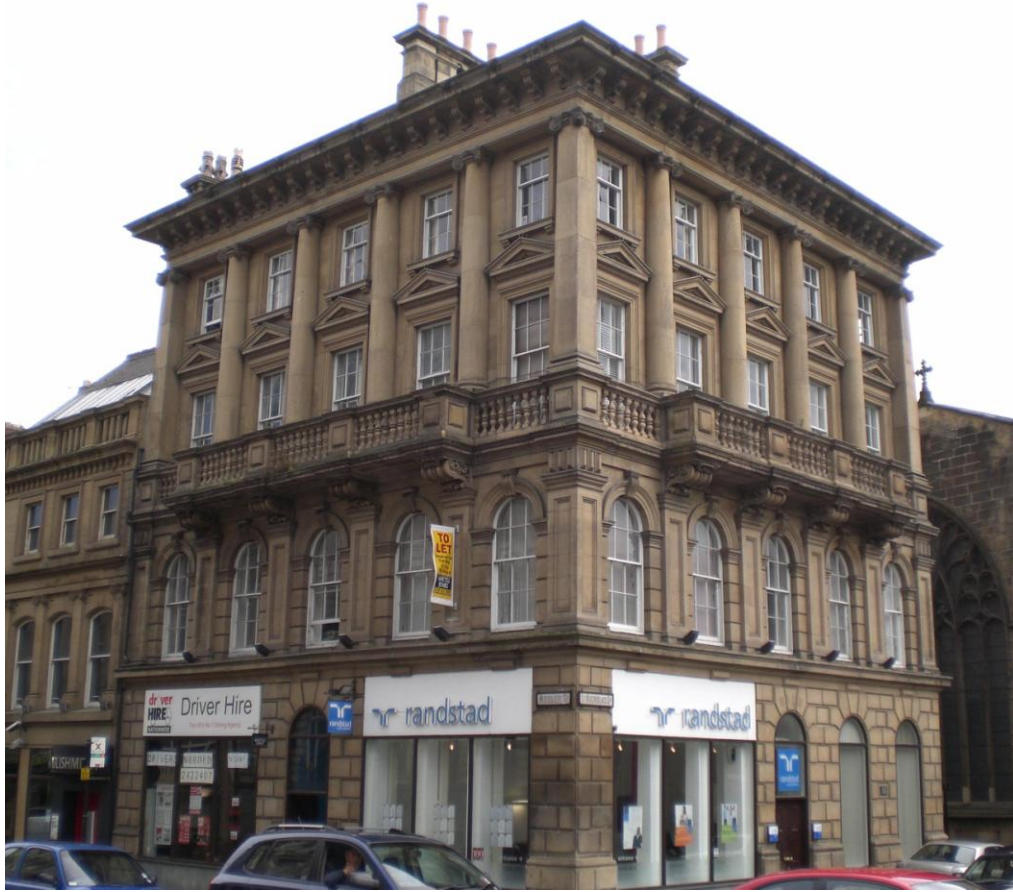
Figure 84 Newcastle Joint Stock Bank, Nos. 40-44 Mosley Street, designed by Benjamin Green, c.1845. (Author's photograph).
