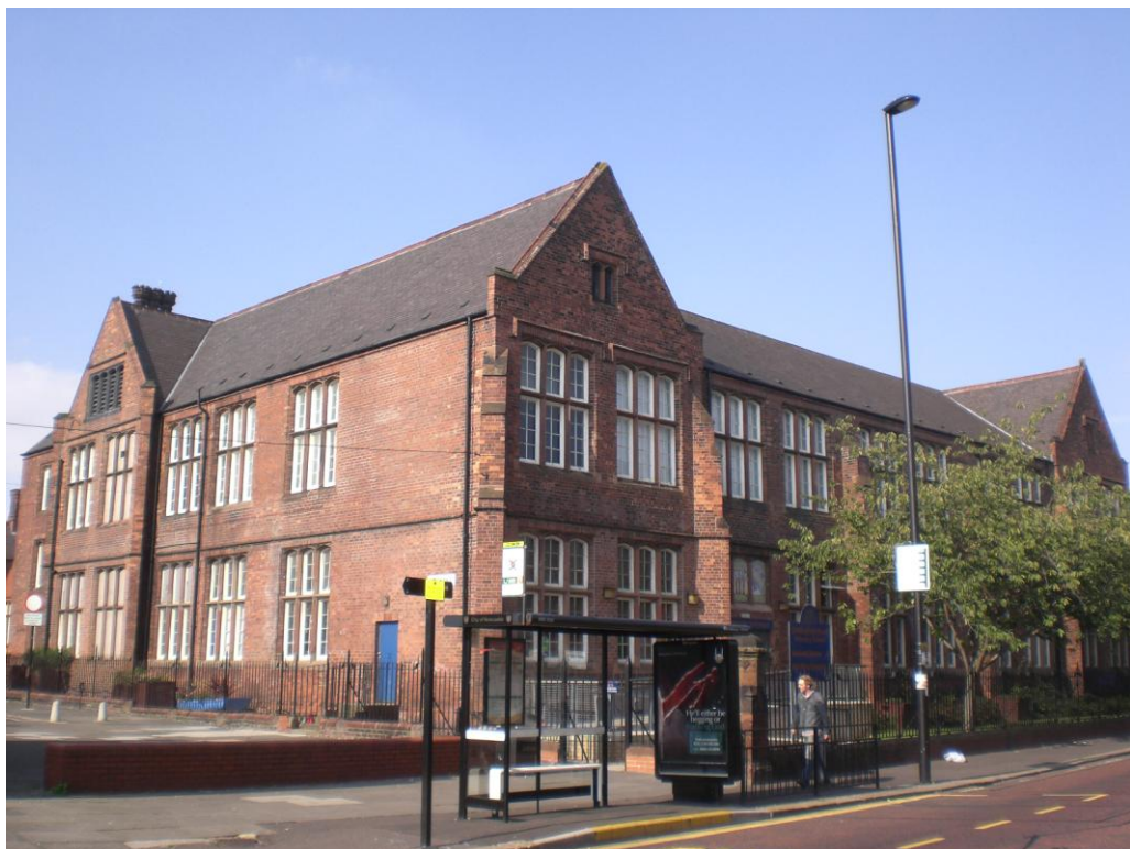
Figure 160 Chillingham Road Board School, designed by Oliver and Leesons, 1893. (Author's photograph).
