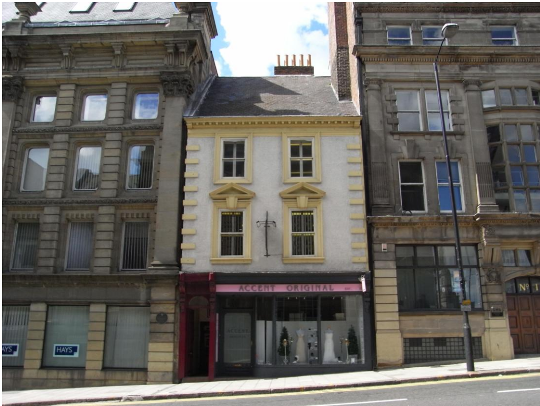
Figure 79 Nos. 3-5 Mosley Street, built as a house and shop, c.1785. (Author's photograph).
