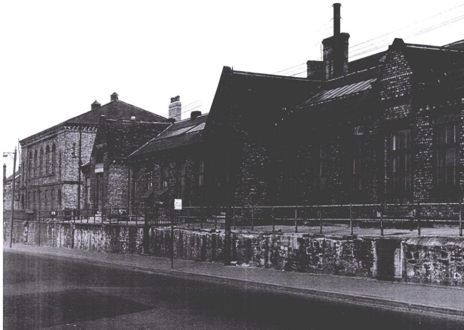
Figure 62 Elswick Works Elementary School in 1972. (Newcastle City Library).
