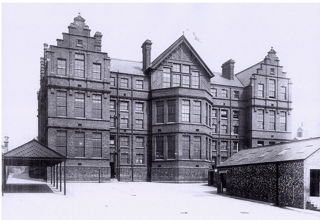
Figure 11 Elswick Road Board School. A covered playground is visible on the left. (Newcastle City Library).
