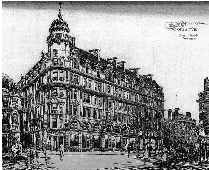
Figure 95 Preliminary design for Collingwood Buildings by Oliver and Leeson. ( The Builder , vol.75, 8 October 1898).
