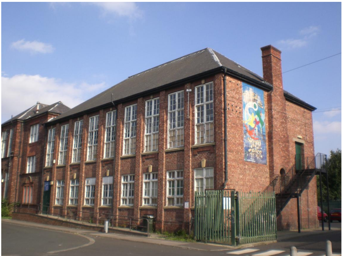
Figure 6 Raby Street Board School, Byker, designed by W. L. Newcombe, 1895-7. (Author's photograph).
