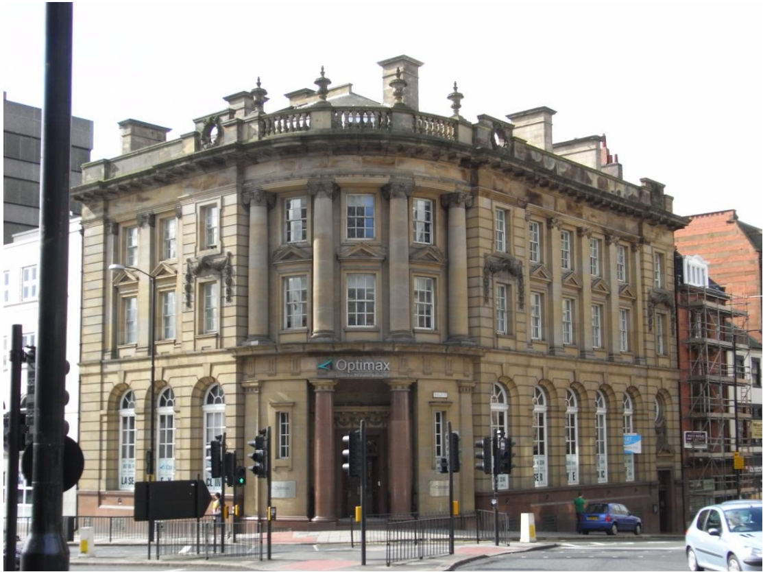
Figure 106 Alliance Assurance Company offices, Nos. 2 and 4 Mosley Street, designed by Newcombe and Newcombe. (Author's photograph).
