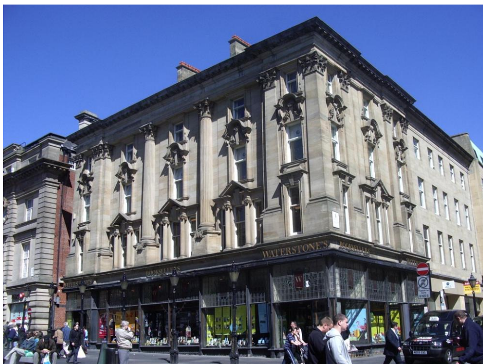
Figure 150 Mawson, Swan and Morgan's Grey Street premises, designed by W.H. Knowles and T.R. Milburn, 1904. (Author's photograph).
