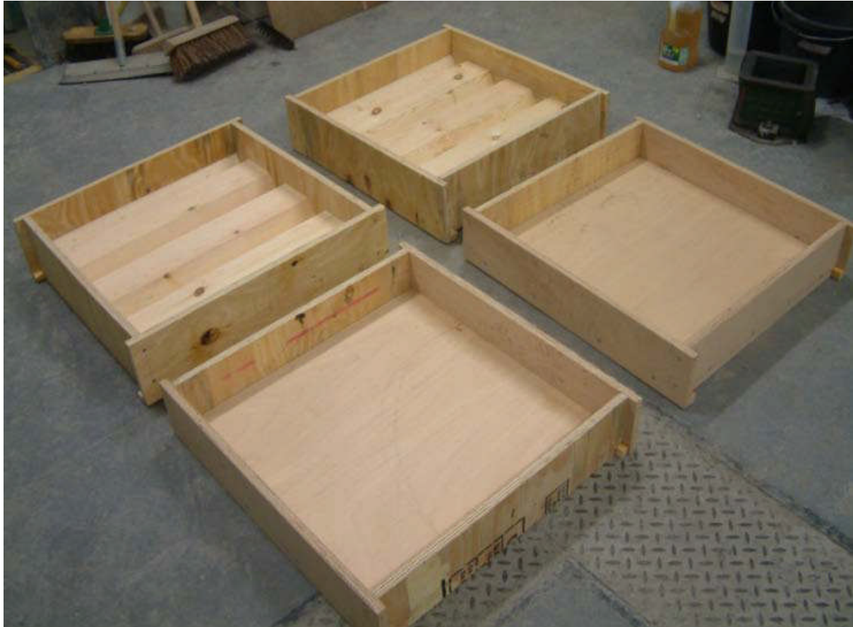
Figure 2: Formwork for test slabs.
