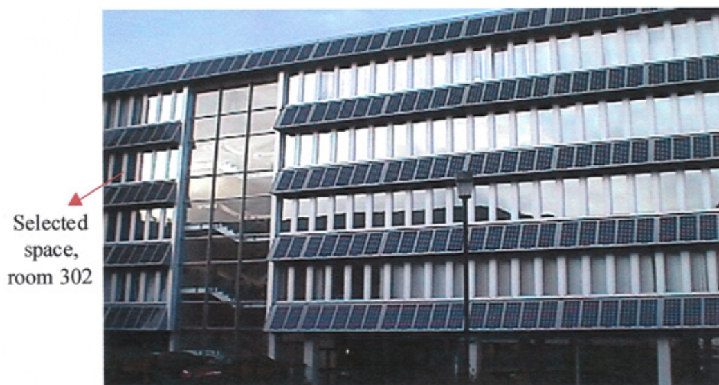
Figure (3.6): Northumberland building, south facing.
