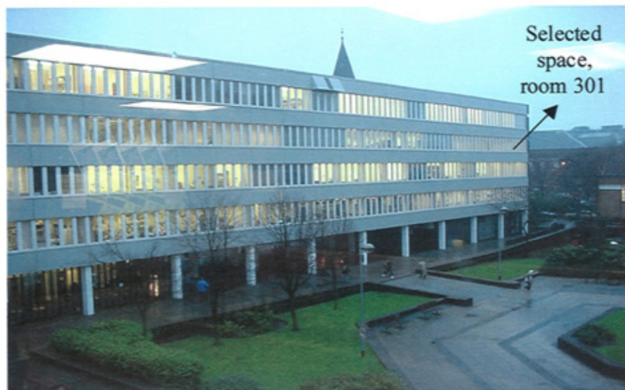
Figure (4.9): Northumberland building, north facing
