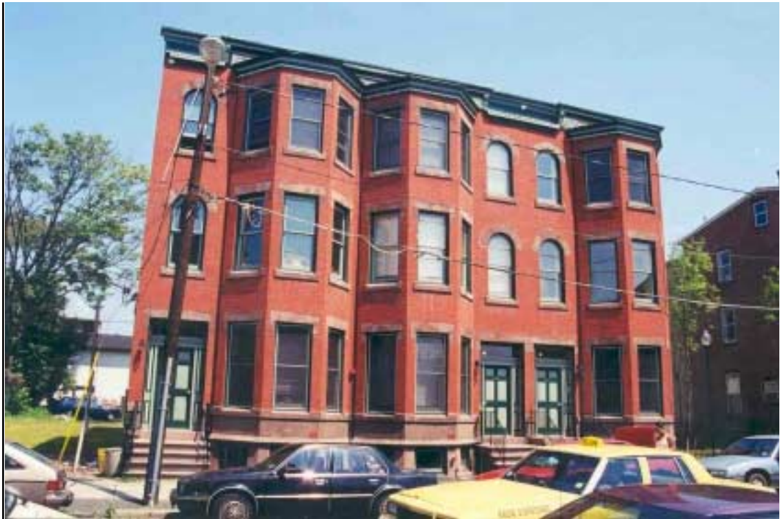
Figure 6: Rehabilitation of No. 210 Academy Street, Trenton, New Jersey (Academy Hanover Historic District): a timber frame and brick residence, constructed in circa 1900. The project involved the conversion of a single residence to two low-income residential units with the assistance of the both 20% federal historic rehabilitation tax credit and the low-income housing tax credit.
