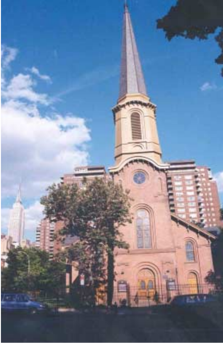
Figure 9: Holy Apostles Church, 9th Avenue and 27th Street, New York. The right to develop air space was transferred enabling the safeguarding of this church.
