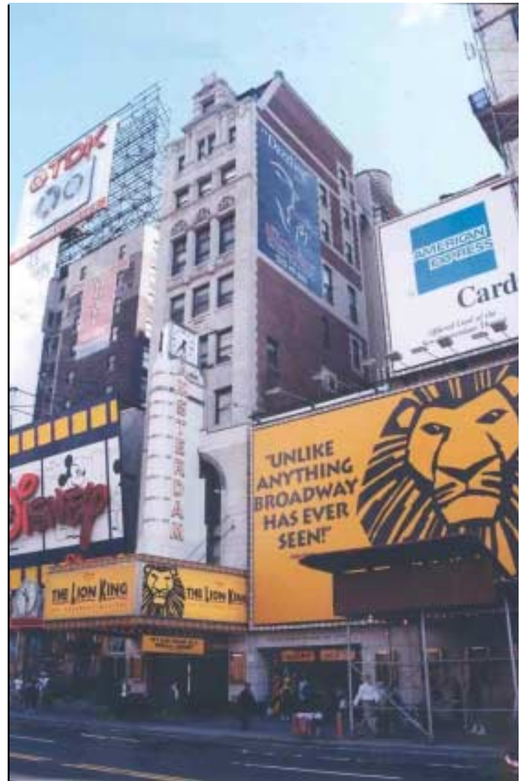
Figure 2: The New Amsterdam Theatre, Time Square, 42nd Street, New York designed by Herts and Tallant in 1903 and listed on the National Register of Historic Places. By the Early 1980s the building was vacant and in a state of disrepair. In 1997 the Disney Development Corporation completed the rehabilitation of the theatre, which involved cleaning and repairing exterior details and restoring the Art Nouveau interior finishes. The total rehabilitation costs eligible for federal credit amounted to $37,100,000 allowing a 20% tax credit of $7,420,000.
