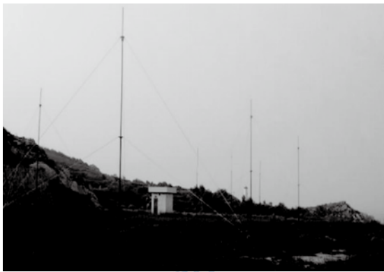
Fig. 1 Antenna array field of HFSWR OSMAR071
