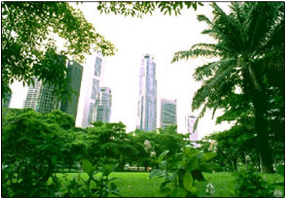
Figure 5.8 Skyscrapers amidst Singapore's 'clean and green' environment depict economic and political stability
