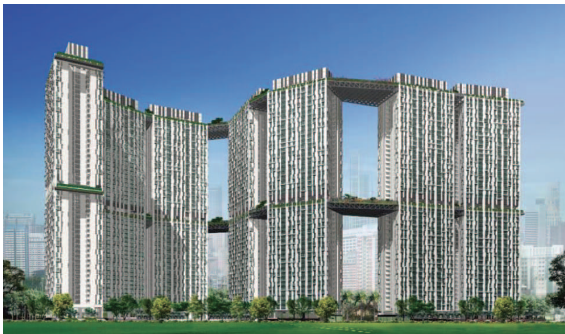
Figure 2.37 The fourth era of Singapore's post-Independence development – the HDB residential estates of year 2000 and beyond can be represented by Pinnacle@Duxton development completed in December 2009
