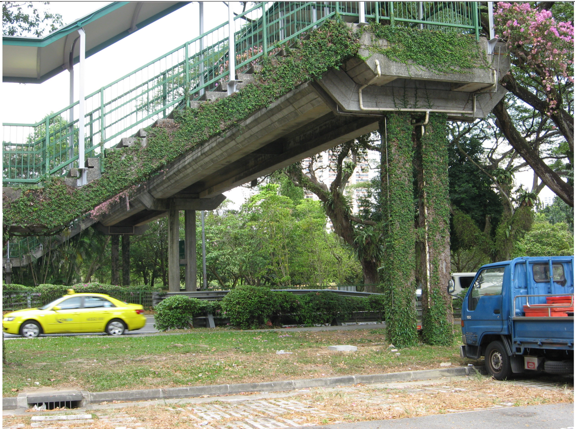
Figure 4.3 Concrete overpass covered with creeping fig vine
