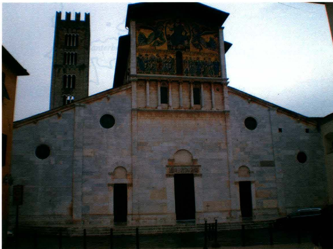
Figure 4: Exterior view of San Frediando, Lucca
