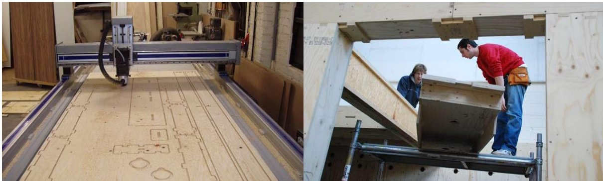
A CNC router used to create prefabricated modules (left, and the modules being assembled on site (right) (Goodeven, 2010)
