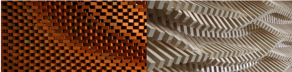
Brick (left) and timber (right) walls assembled by a robotic arm (Gramazio & Kohler, 2010)
