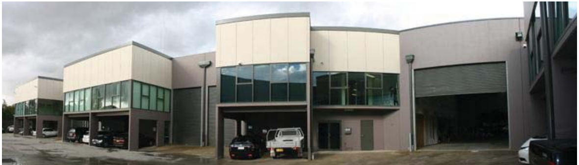
Figure 3.8 The case study building façade facing north.
