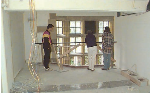
Building a mezzanine
