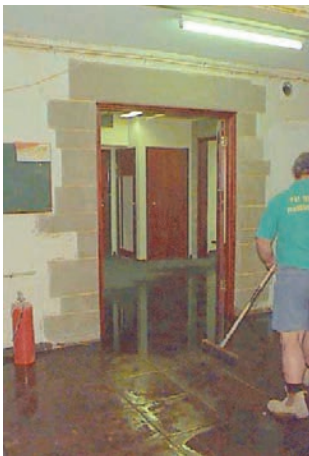
Flood in the foyer
