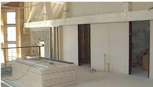
Constructing a mezzanine
