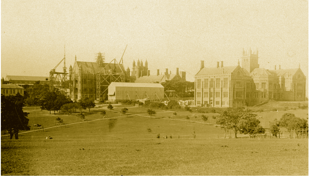
Building the south-west corner of the Quadrangle, later the Fisher Library and more recently MacLaurin Hall. The original (south) wing of the Anderson Stuart Building is on the right.
