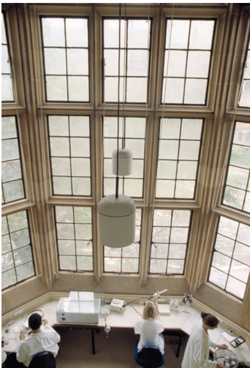
Refurbished laboratory with mezzanine floor, preserving the depth of the windows framed in sandstone
