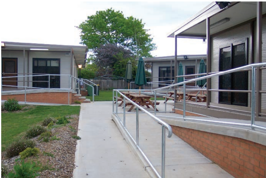
Student accommodation at Orange
