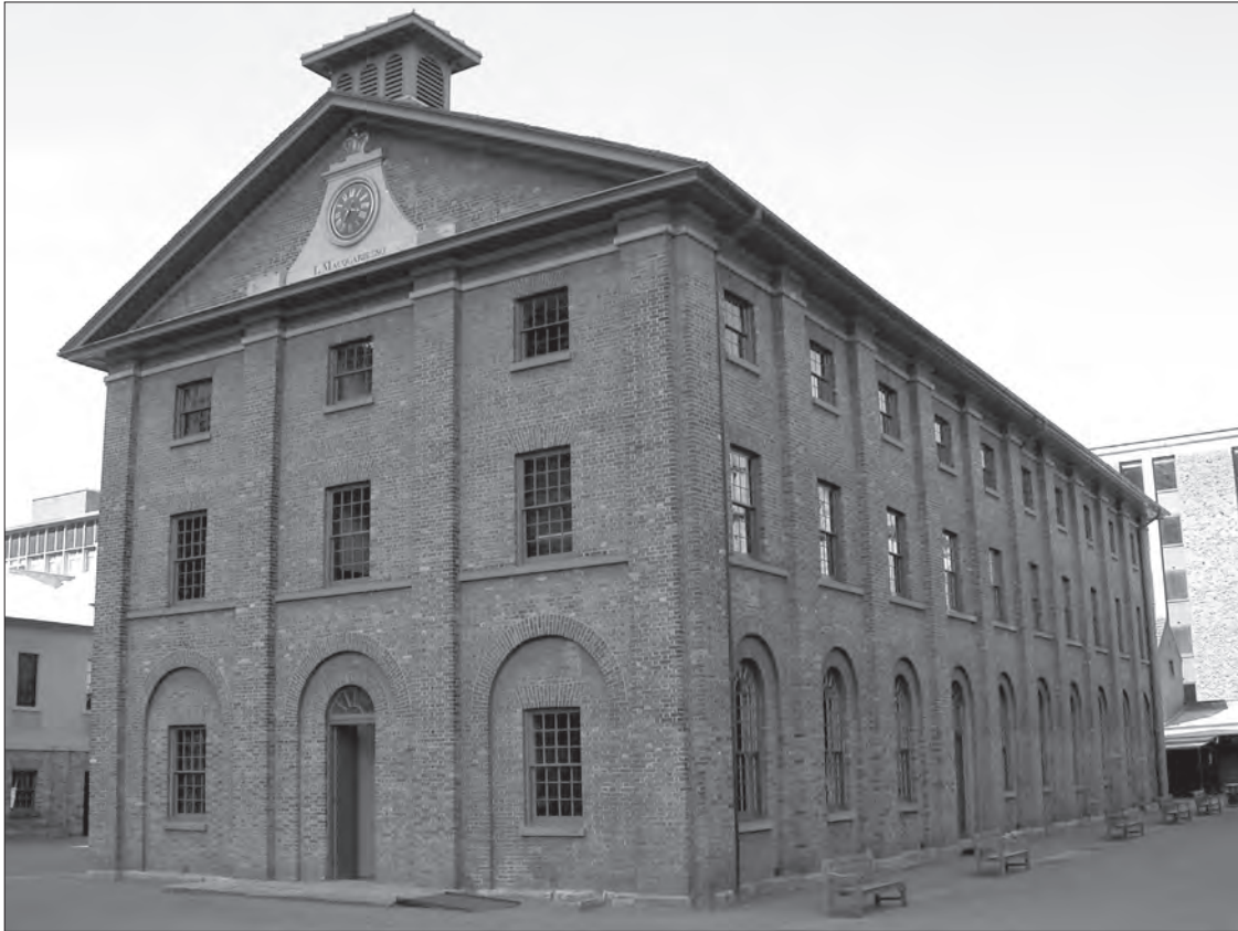
Figure 1.4: General view of Hyde Park Barracks main building (P. Davies 2008).
