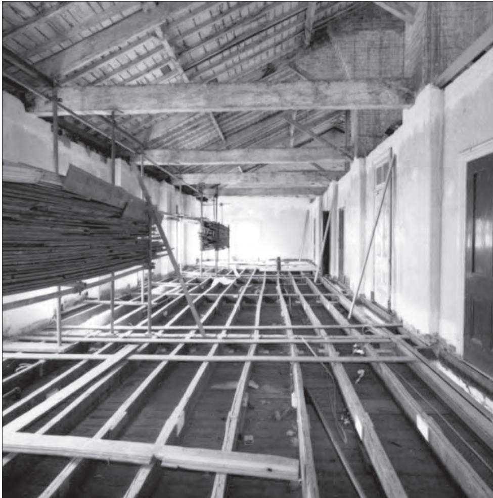
Figure 2.1: Cavity spaces between the joists below the floor on Level 3, looking east. Note the stack of floor boards on the scaffold at left (V. Pavlovic 1982).
