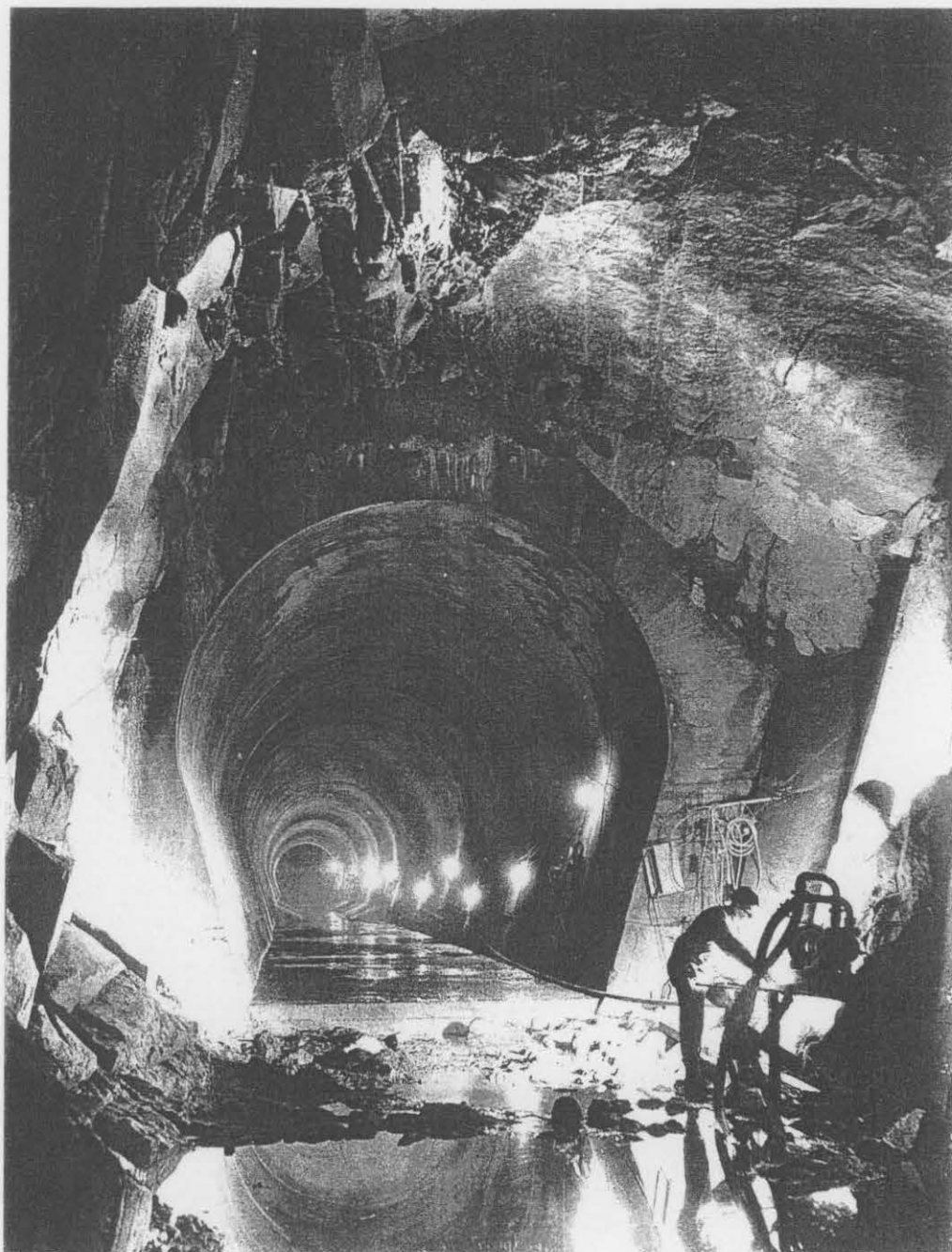
76 GUTHEGA Looking downstream towards the surge chamber in Guthega Tunnel.
