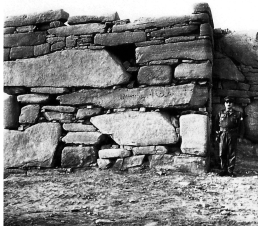
Figure 5.16 - Masjed-e Soleyman. Substructure wall (Ghirshman 1976, Pl. LII, 2).
