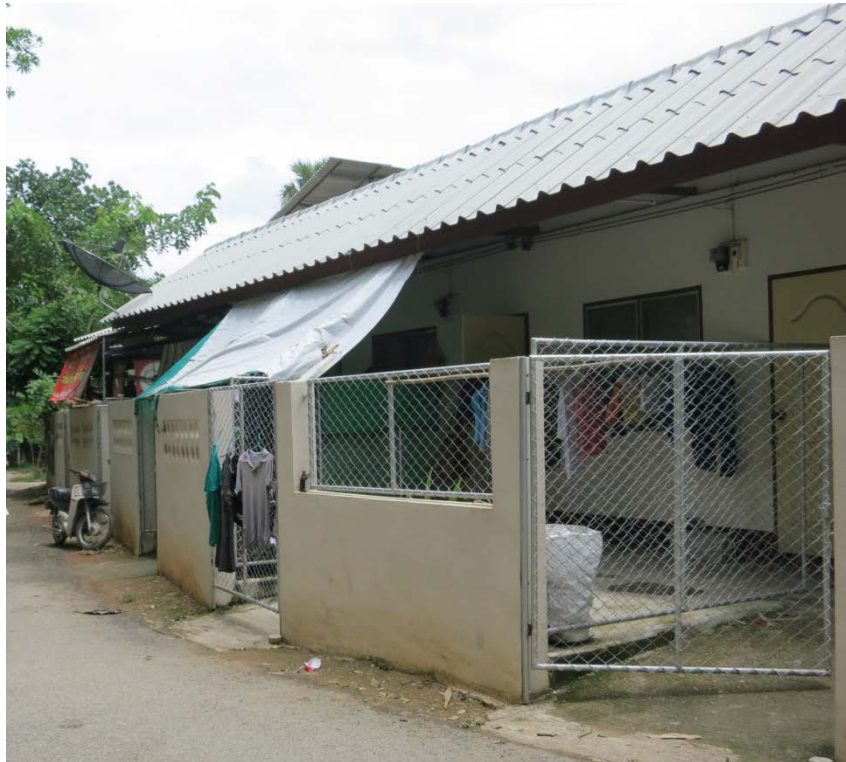
Figure 4.19: The most recent 5 unit dormitory in Nam Jam, 2011 (July 2013)
