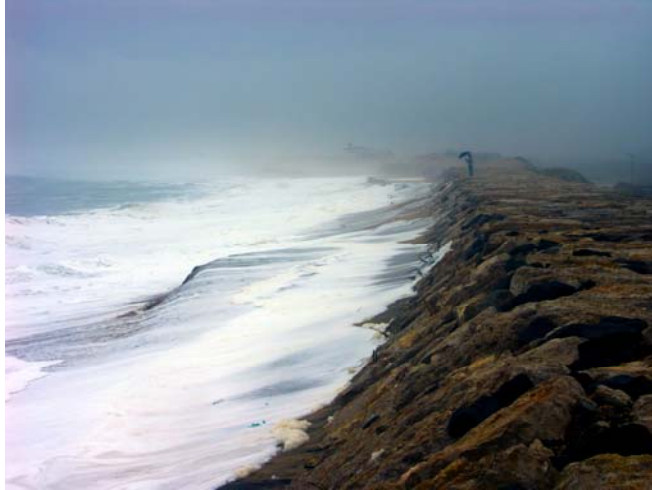
Figure 5.26 - Sea-wall structure composed by loose rocks in the northern part of the northern sub cell, constructed under emergency conditions when severe storms threatened urbanized areas in 2007.
