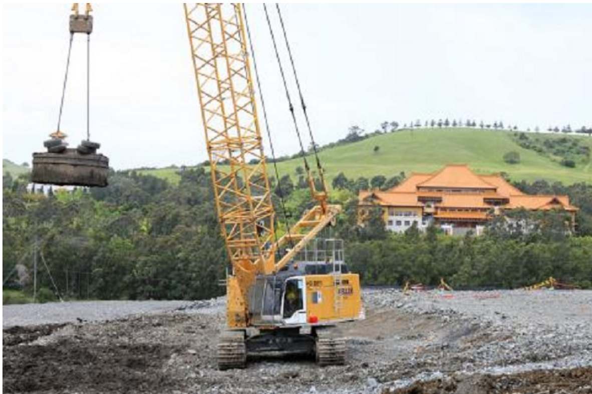
Figure 1.1. Dynamic compaction equipment- crane and tamper (courtesy of Keller Australia).
