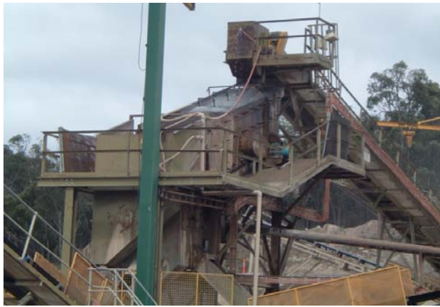
Figure 133: Marulan quarry crusher and washer
