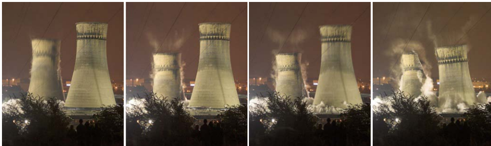
Plate 6. Destruction of Tinsley Cooling Towers [Siandara (2008)]
