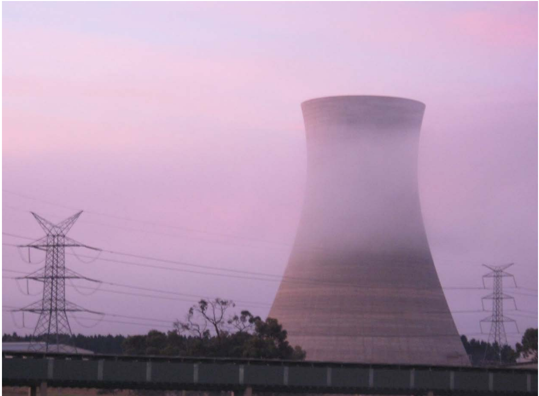
Plate 7. Wallerawang, NSW cooling tower
