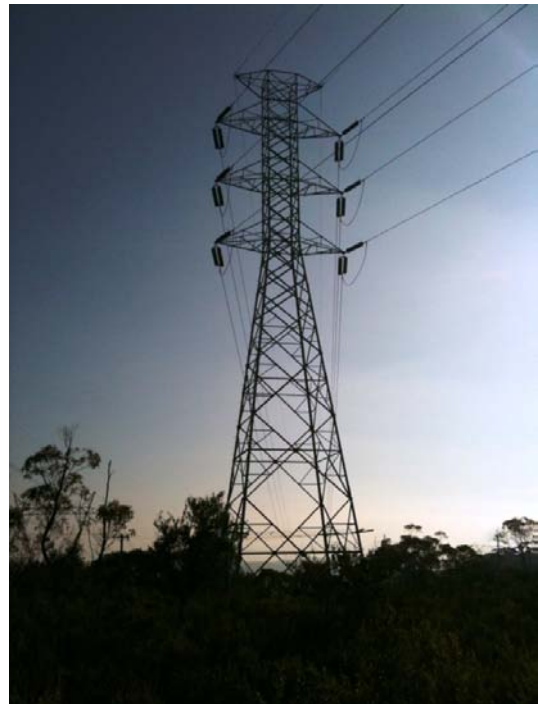
Plate 11. Pylon at Sherbrook, NSW.
