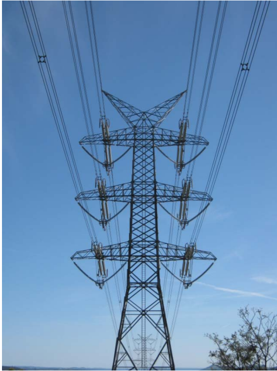
Plate 8. Pylon at Wallerawang, NSW.
