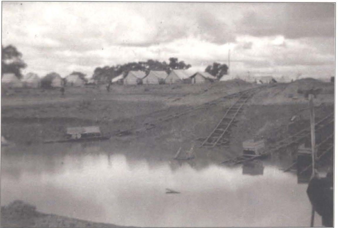
Railway Reservoir on Warioota Creek
