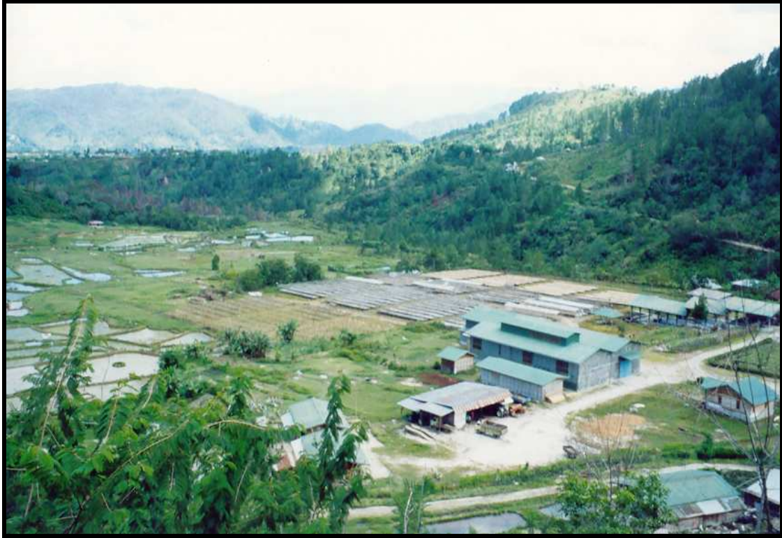
Plate 7-17 Processing plant and sun-drying facilities, Sulutco Jaya Estate, Bolokan Village
