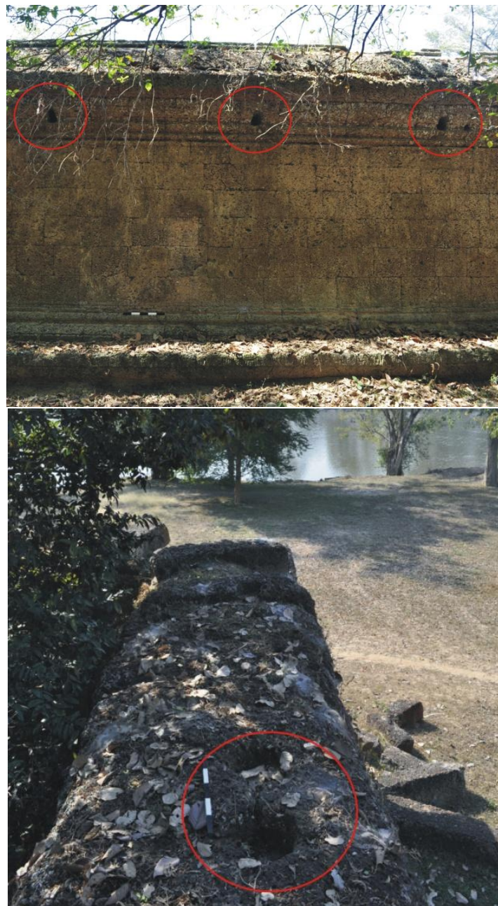
Figure 1.5 – Postholes in the fourth enclosure wall: horizontal on the inside face (above) and vertical on top (below)
