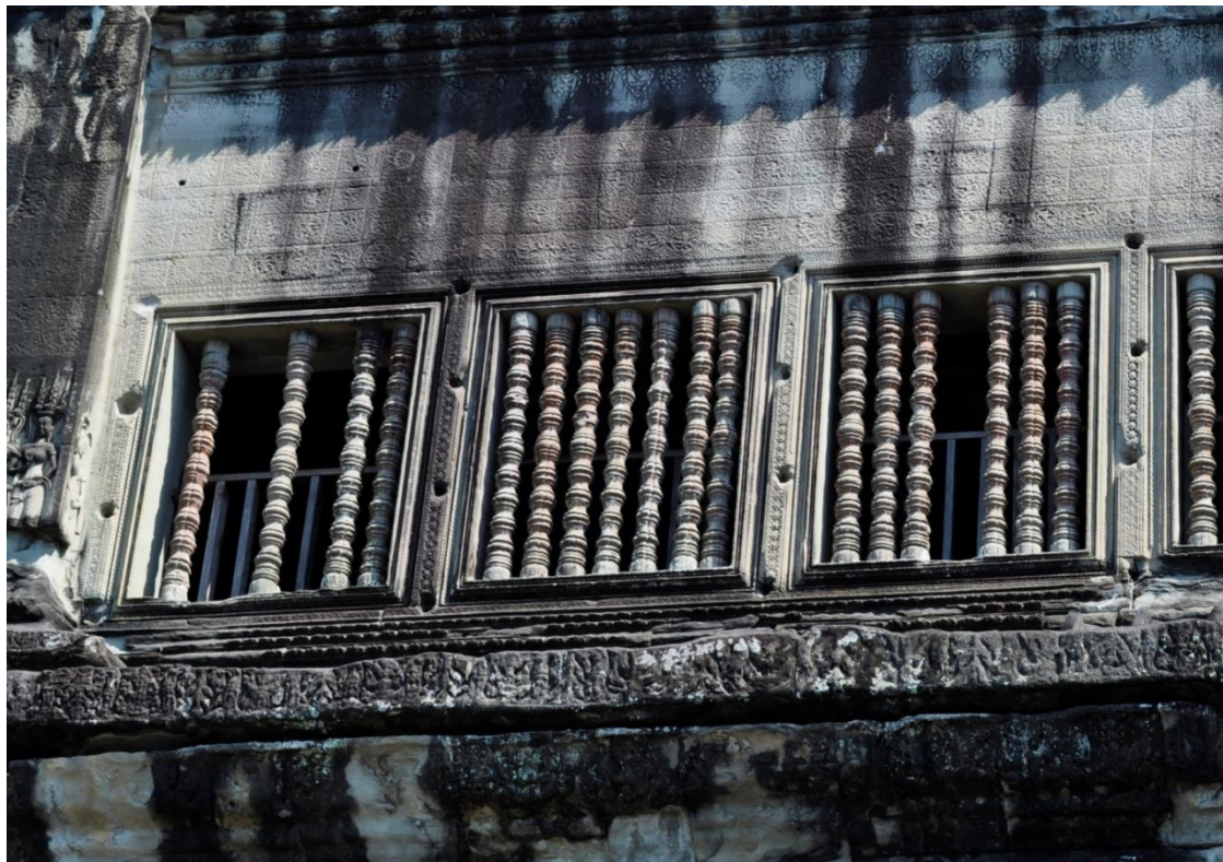
Figure 1.4 - Postholes on the outside of the central enclosure of Angkor Wat - Note how they interrupt the decorative pattern
