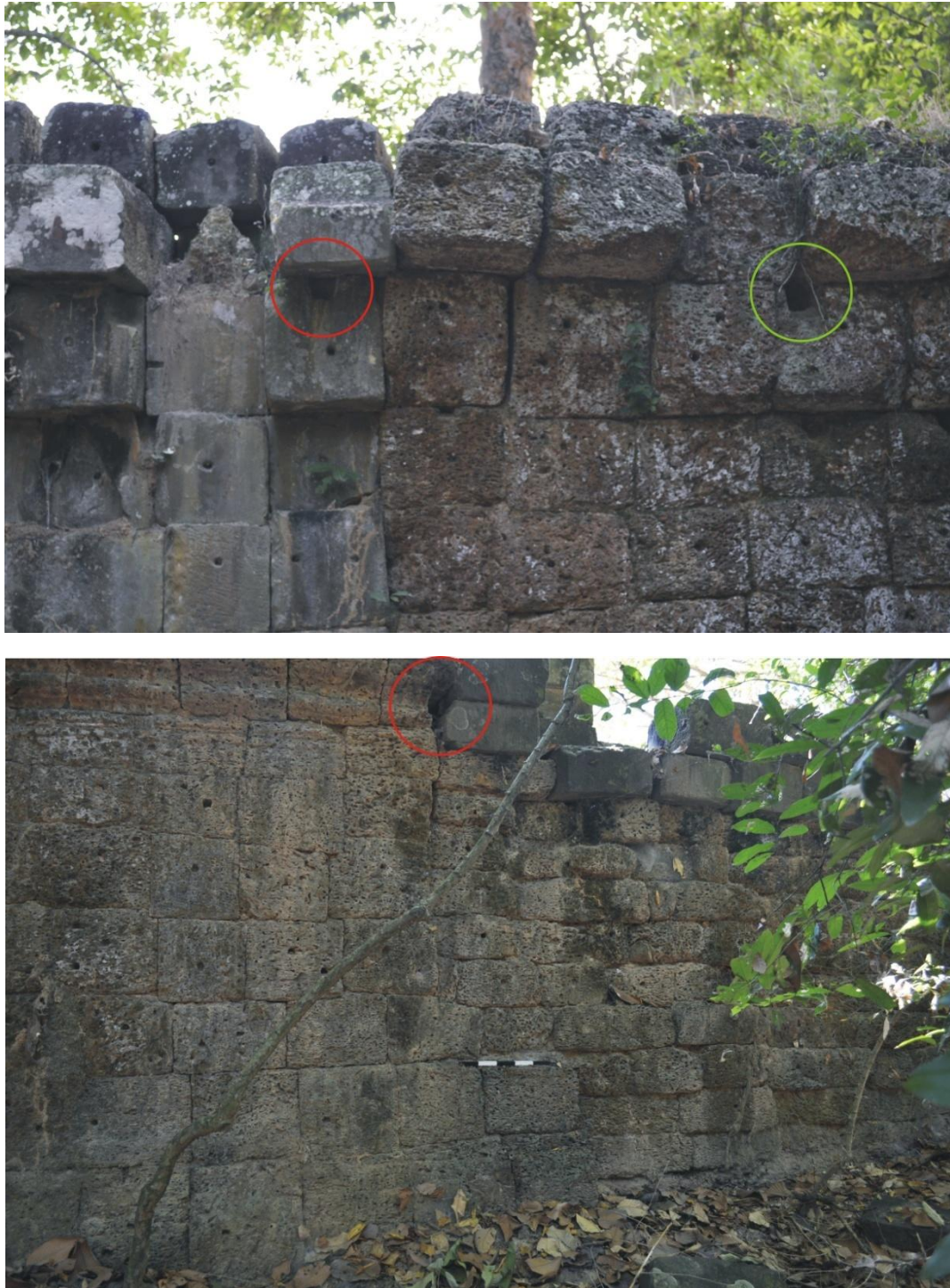
Figure 5.30 – Horizontal postholes in the original wall (green) and the later modifications (red) – South wall, East gateway (above), South wall, West gateway (below)
