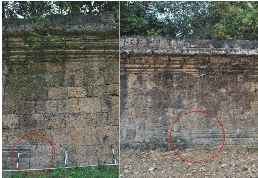
Figure 4.27 - Changes in surface finish detail in the South wall, West sector, exterior, near the West gateway –West of the gateway (left) and East of the gateway (right)
