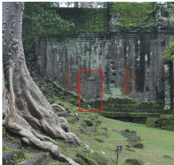
Figure 7.4 - West wing of the North gopura, interior. Blocked up doorway highlighted.
