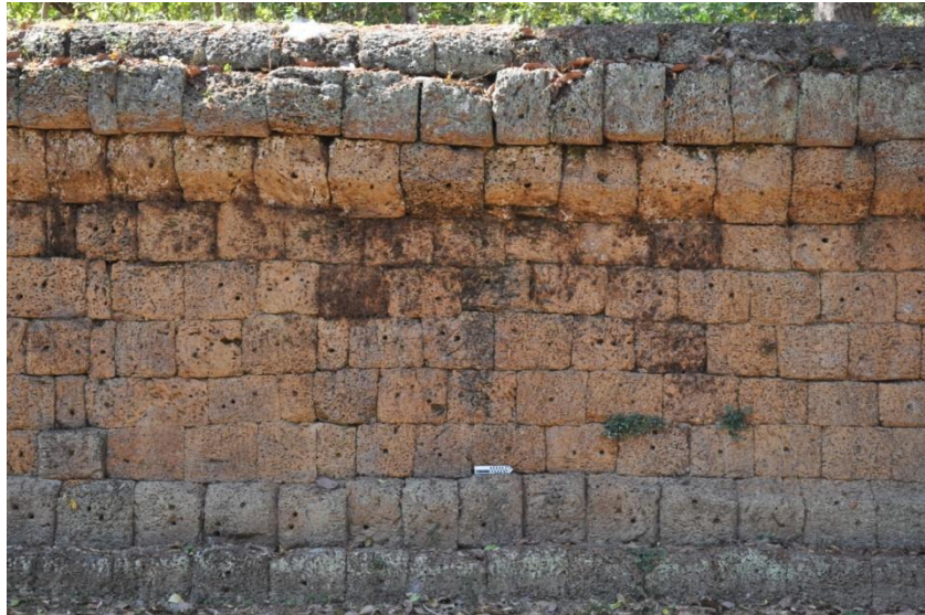
Figure 4.5 - Manoeuvring holes in the exposed face
