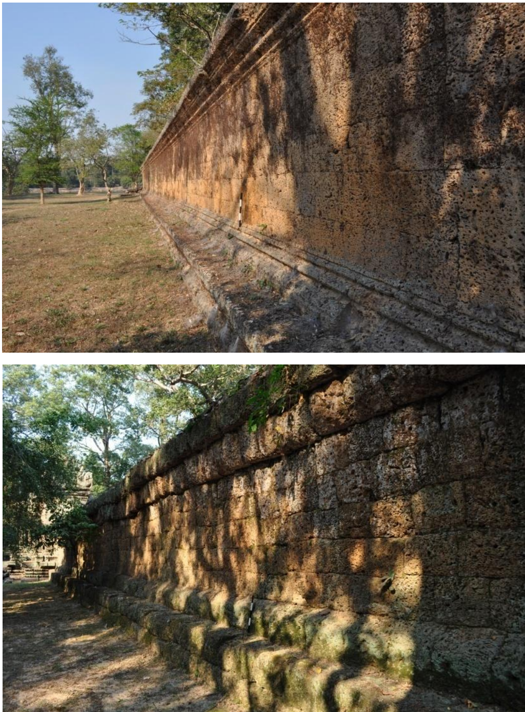
Figure 4.14 The difference in surface finish between the West half (above) and the East (below)
