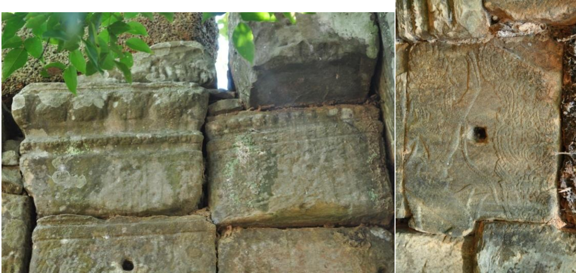
Figure 5.28 – Decorated blocks recycled in the North wall, East gateway: left – pillar cornice blocks (exterior), and right – dancing apsara (interior)
