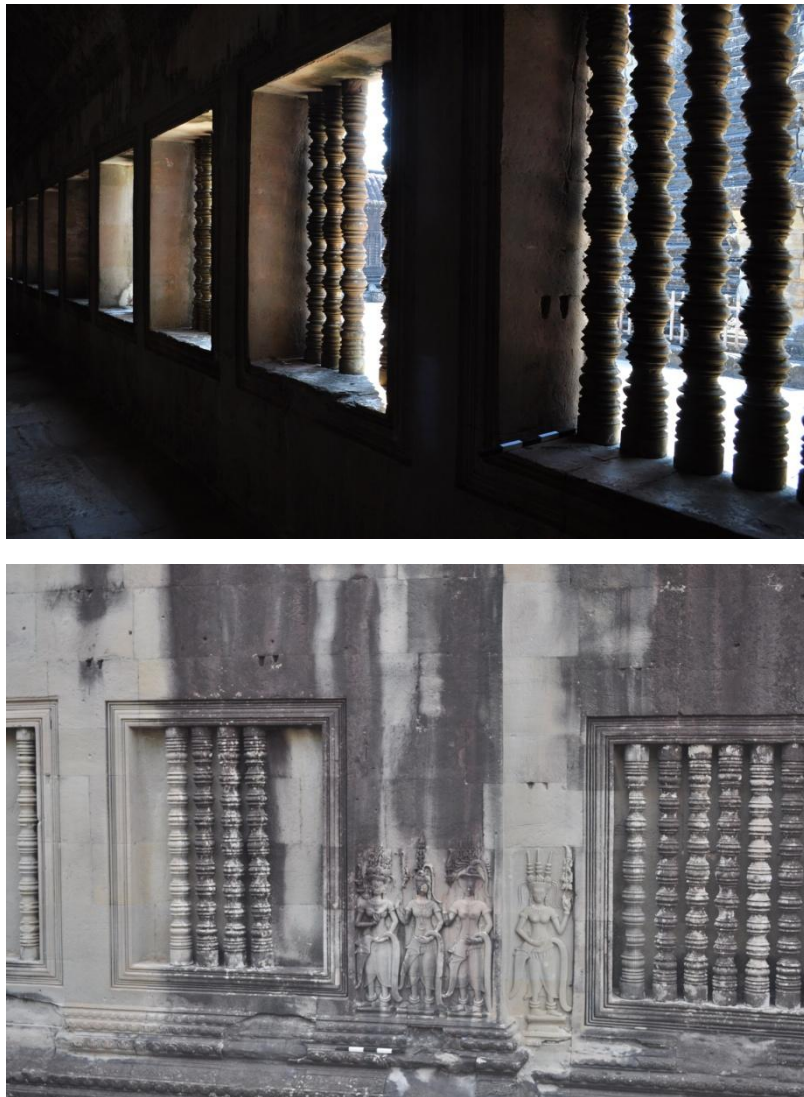
Figure 3.4 Real (above) and false (below) balustered windows in the inside wall of the second gallery
