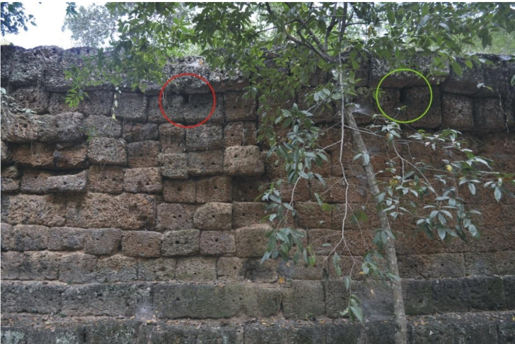
Figure 5.29 - Horizontal postholes in the original wall (green) and the later modifications (red) –North wall, East gateway (above), East wall, North gateway (below)
