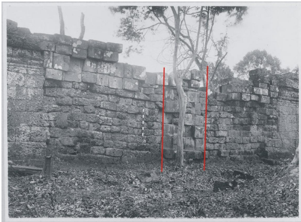
Figure 5.26 – South wall, West gateway, showing the pattern of laterite and sandstone components (EFEO archives)
