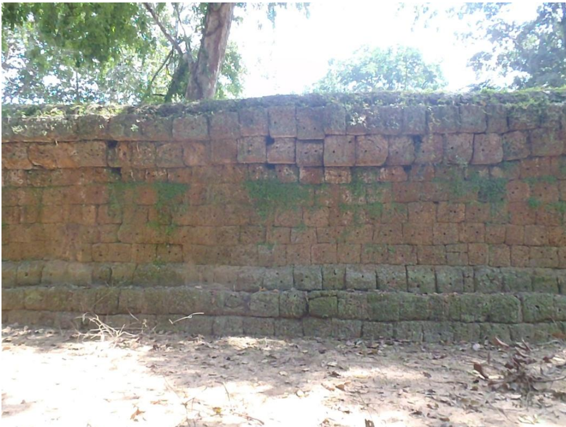
Figure 5.8 - Postholes forming parallel lines: East wall, South side, near the East gopura.
