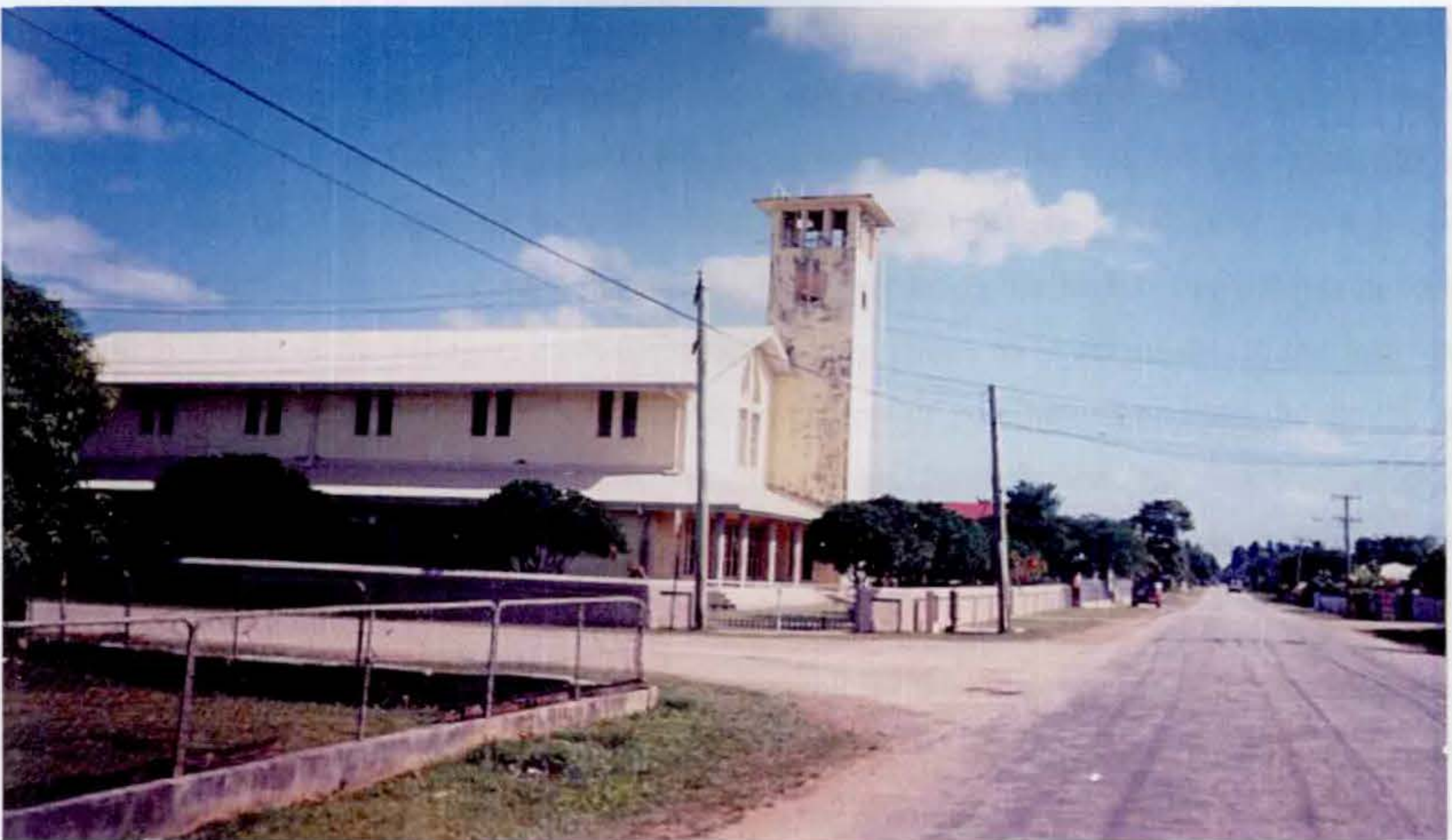
Figure 5.7 FWC building in Nukunuku.
