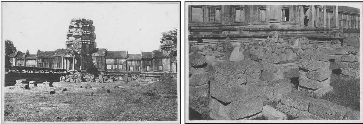
FIG. [59]: COLUMN BASES EXCAVATED BY PARMENTIER & MARCHAL, 1919/1920 (SOURCE: EFEO ARCHIVES No. 05393).
