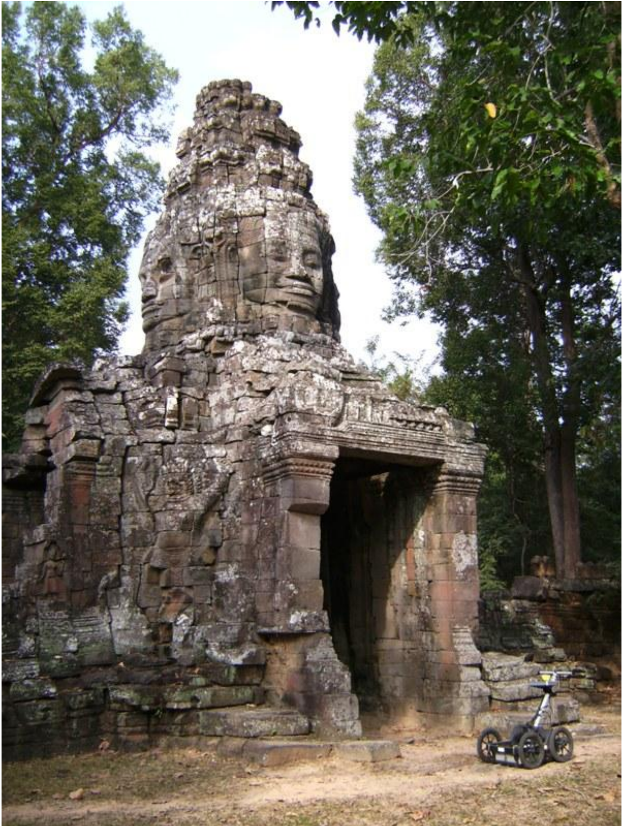
FIG. [1]: THE GPR CART IN FRONT OF THE SOUTH GATE OF BANTEAY KDEI.
