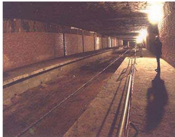
Figure 2 annex 3.2: Sevilla Metro tunnel
