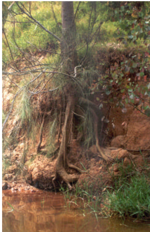
Figure 3.16: A 10 m tall Casuarina tree growing within the study area. Substantial roots are visible growing into the bank material at a depth of 1.6 m below the ground surface.
