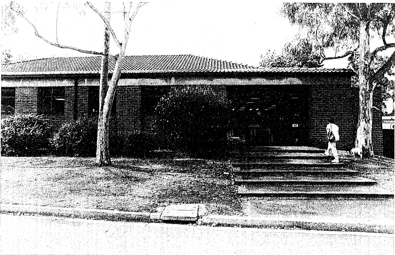
Evelyn Williams Building — Veterinary Teaching Hospital
