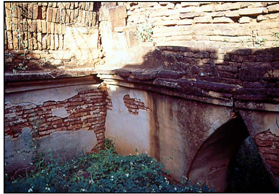
Figure 124 Gu Gyaung temple, detail of interior brickwork.
