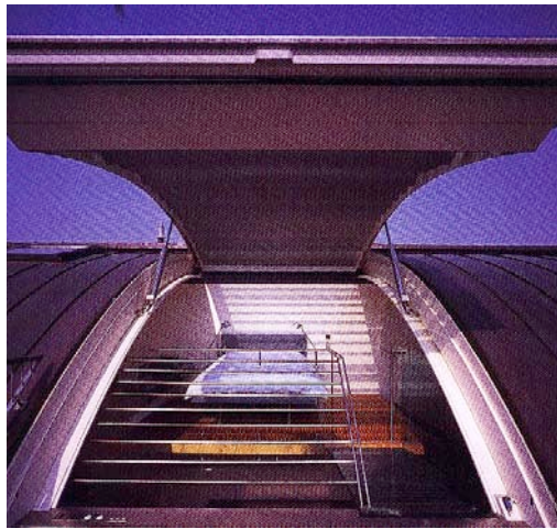
Plate 4.18 A roof-door — the ultimate in Unbound skylights, London
