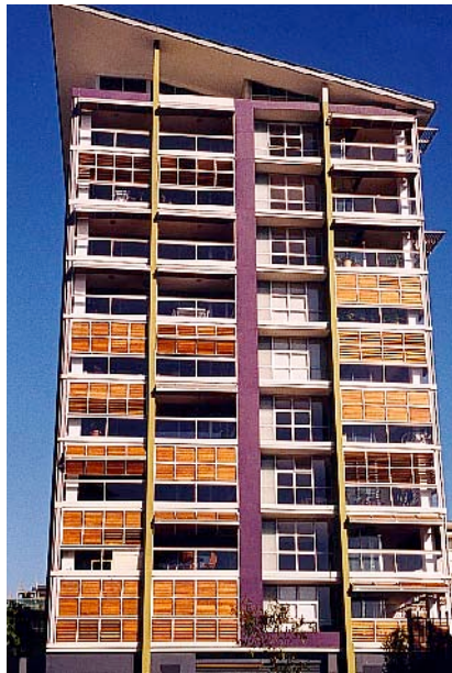
Plate 4.110 Wooden louvres, inner city apartment block, Sydney
