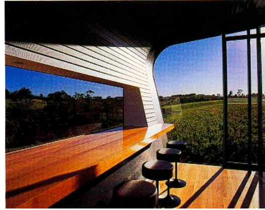
Plate 4.114 Outward and forward sloping wall
