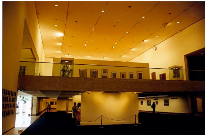
Plate 4.37 A suspended slab, Queensland Art Gallery
