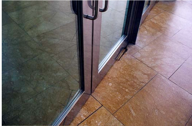
Plate 4.48 Continuity in exterior and interior flooring, Guggenheim Museum, Bilbao
