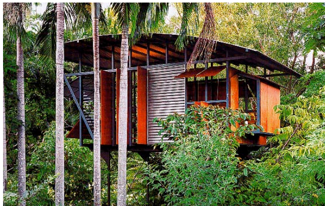
Plate 4.28 Floating roof in Australian tropics
