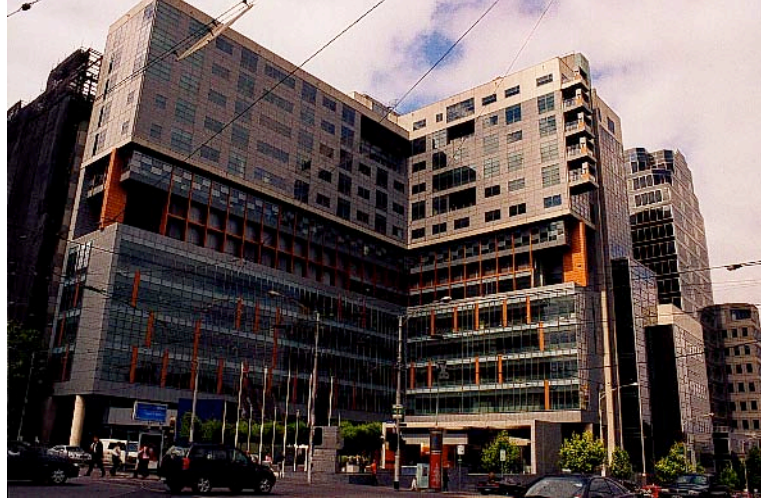
Plate 3.35 The Commonwealth Law Court building, Melbourne
