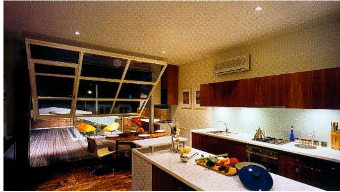
Plate 4.109 Visual and physical diaphany — a lift-up wall panel
