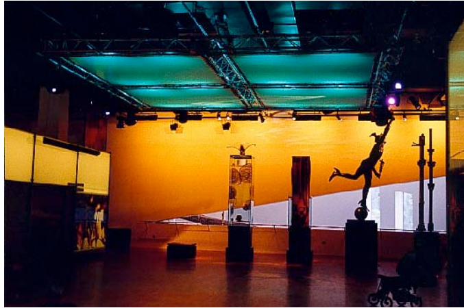
Plate 4.27 Adjustable ceiling, performance space, Australia gallery, Melbourne Museum
