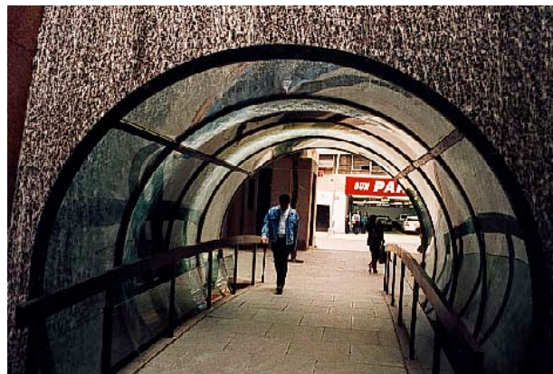
Plate 4.91 Pedestrian tunnel, New York
