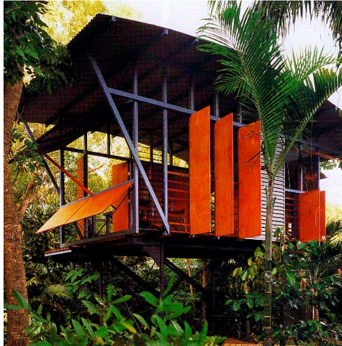
Plate 4.112 Vertical and horizontal ventilation gills
