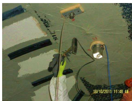
Figure 13. Sledge hammer applied to the crown of the vault intrados.
