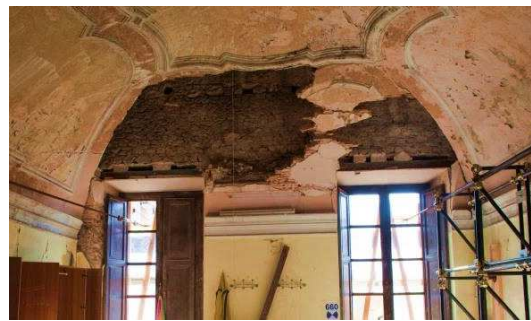
Figure 3. The thin vault tested in the city of L'Aquila.
