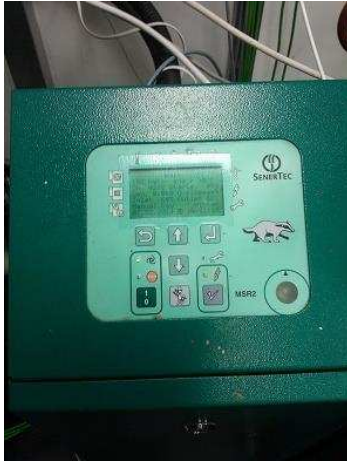
a) The digital display of the unit to monitor key parameters of the mCHP operation
