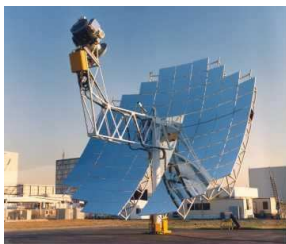
Figure 2.8 A 25 kW tracking, concentrating solar power (CSP) dish collector [6]
