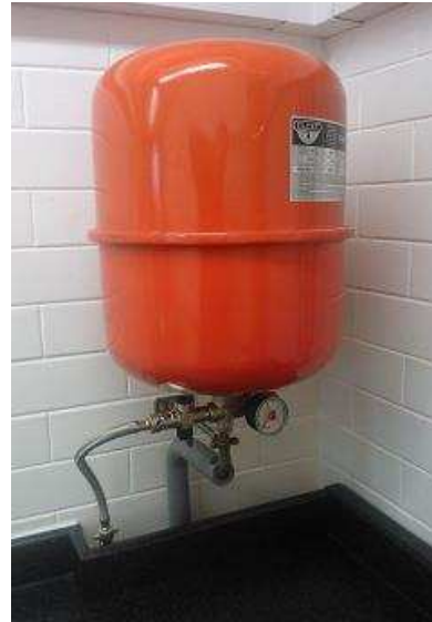
b) Pressurisation vessel to maintain constant pressure in the hydronic circuit
