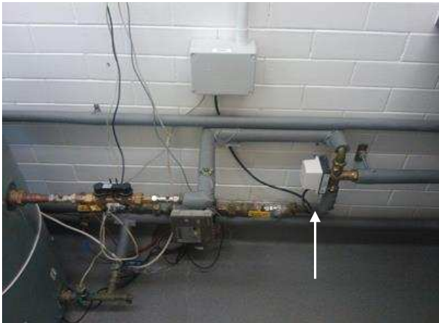
c) White arrow points to the 3 way valve. The operation of the valve is both temperature and manually controlled
