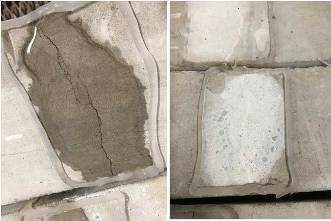
Figure 4 – Cracked concrete beam on left and healed concrete beams to the right.
