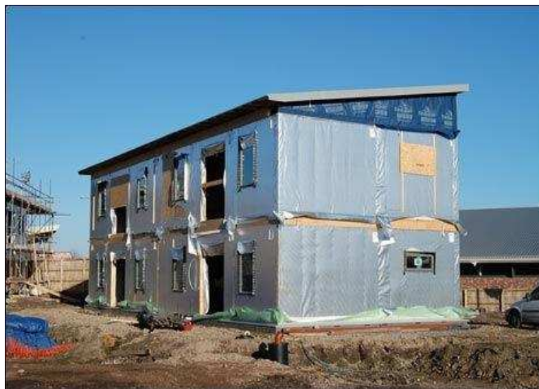
Image 03: BoKlok Generation 1 Apartments timber framing system under construction (Image: D.Morton)
