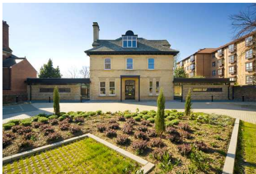
Figure 7.3 Clayton House Renovated
