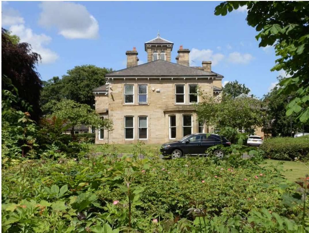
Figure 2.8 Villa development, Fernwood House, Clayton Road
