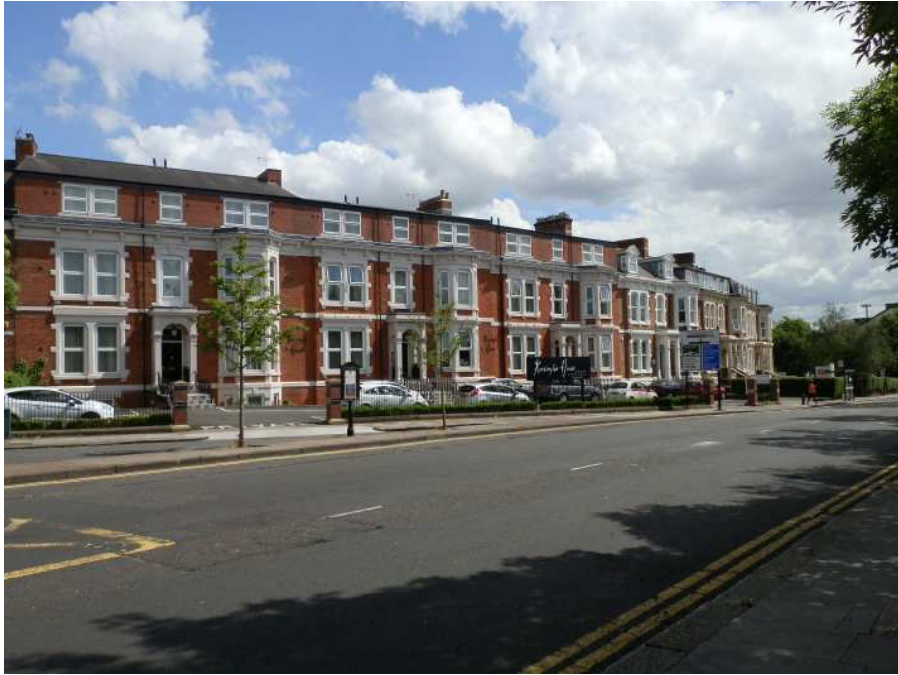
Figure 7.5. Osborne Road. Terrace Restoration
