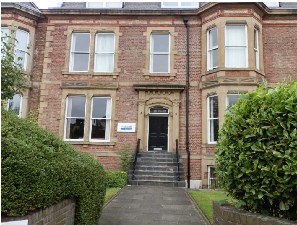
Figure 3.13. Solicitor's Office, Osborne Terrace
