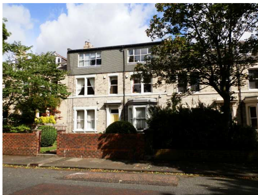
Figure 3.9. Vertical roof extension to create additional residential space, Osborne Avenue
