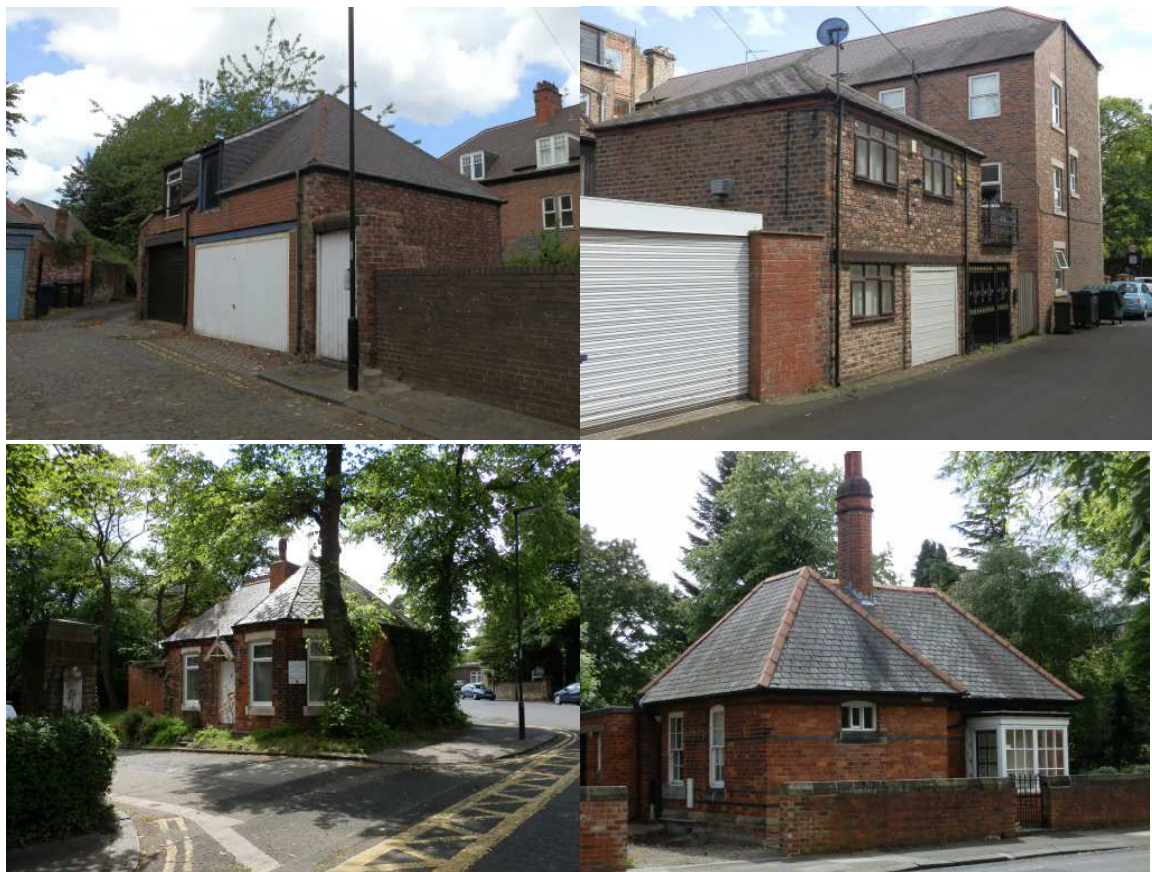
Figure 7.7 Restoration of Carriage Houses and Gatehouses
