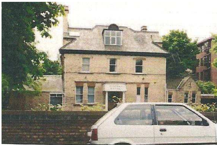
Figure 7.2 Clayton House, vacant in 1990s
