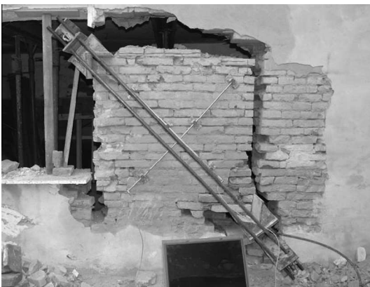
Fig. 1. On-site diagonal compression test (San Felice building).
