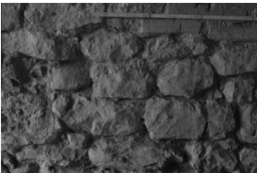
Fig. 7. Stonework of Colle Umberto farm house (20th-century).
