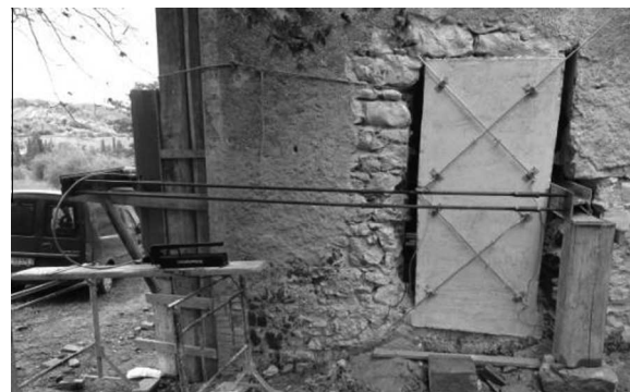
Fig. 2. On-site shear-compression test (Colle Umberto building).
