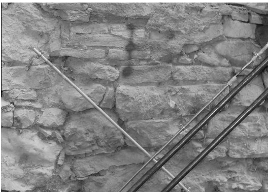
Fig. 6. Stonework of Colle Umberto farm house (19th-century).
