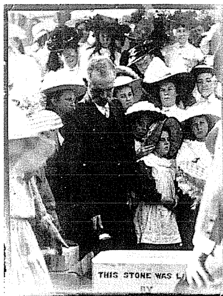
Figure 5: Laying of Mt Eden Baptist Foundation Stone 127
