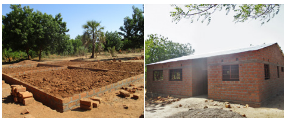
Photo 4-5: The new Lusitu community seed bank under construction. Credit: ZARI
