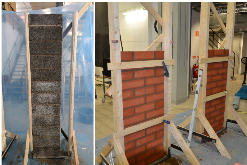
Figure 2.7 Manufacturing of the LWA block walls in series 2 (left); clay brick walls in series 3 (left).
