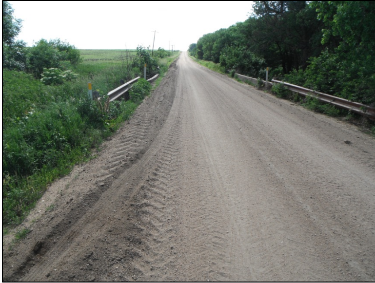
Figure 4.8-4. Sand-and-gravel roads cross Cub Creek and its tributaries frequently throughout the watershed, leading to some deposition directly into the channel at bridge crossings. Photo by Johannes Beebee, Colorado State University.
